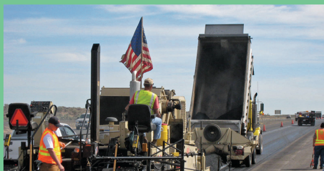
Workers with the Washington State Department of Transportation are using warm-mix asphalt paving for the first time on I-90 near George, WA. Warm-mix asphalt lowers the required temperature for processing at the plant and application at the jobsite, saving energy and cutting air emissions. It also can improve compaction. Photo: Craig Weiland, University of Washington.
