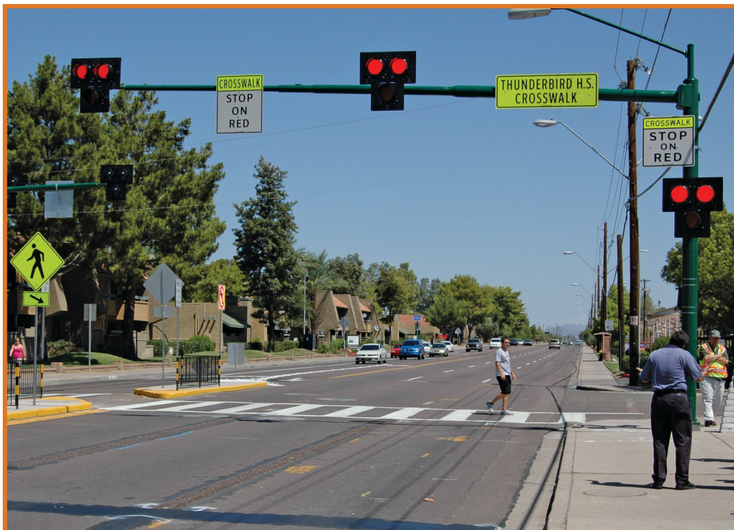
Pedestrian hybrid beacons, such as this one in Phoenix, AZ, provide a break in traffic to allow pedestrians to cross safely. The device is activated when pedestrians engage a nearby pushbutton.
