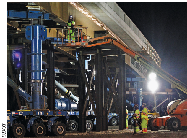
Starting around 2006, the Utah Department of Transportation (UDOT) began erecting dozens of interstate bridges over weekends by implementing ABC as its standard practice. In 2008, UDOT bundled projects together and created this staging area, which local residents nicknamed the “bridge farm.”
