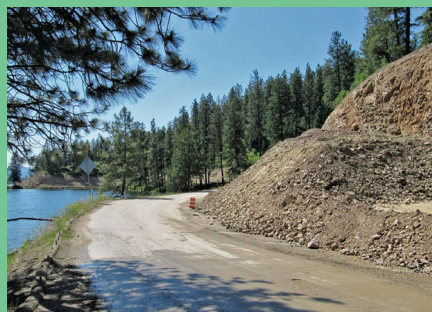
Fernan Lake Road (left) in Idaho Panhandle National Forest is traversed by wildlife (center) as well as vehicles. During construction (right), workers recontoured the steep slopes to better manage stormwater runoff and groundwater recharge.
