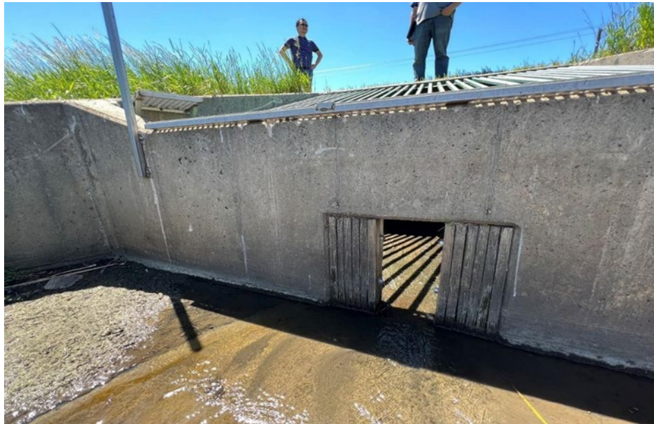
Figure 3.6 The selected stormwater BMP site retention pond outlet structure
