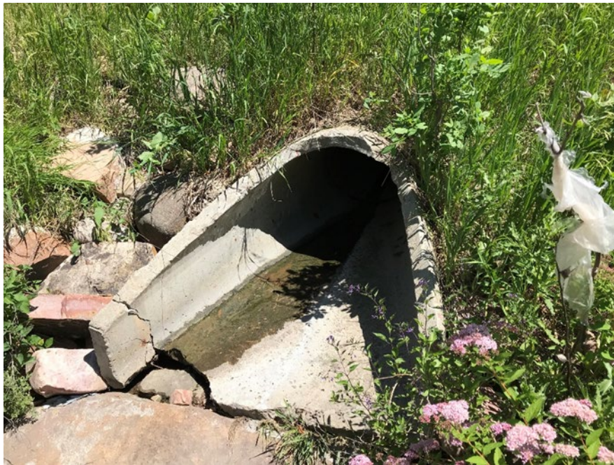
Figure 3.5 Stormwater site 1201 N Sycamore Avenue
