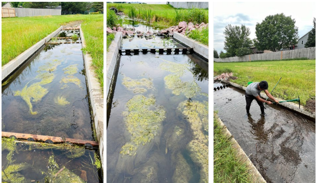
Figure 3.16 Filter structure before and during filter maintenance
