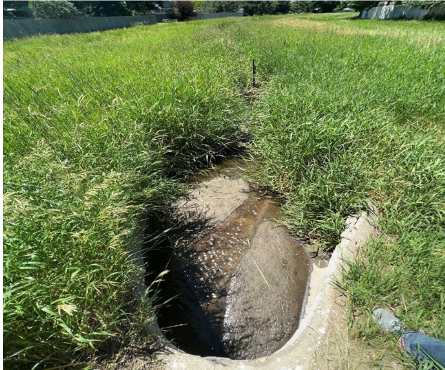
Figure 3.8 The discharge channel inlet structure
