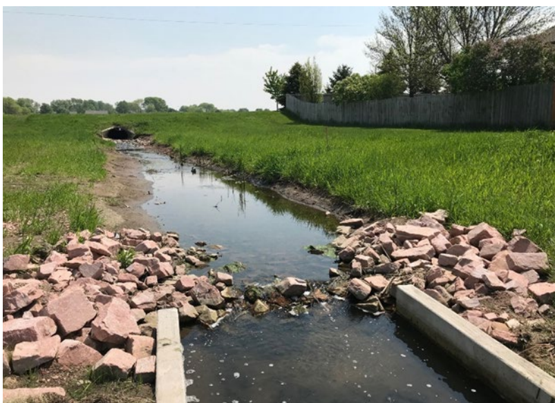
Figure 3.14 Filter structure inlet
