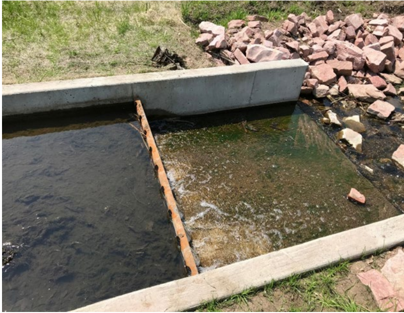
Figure 3.15 Filter structure outlet
