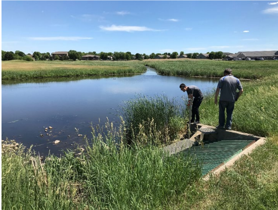
Figure 3.4 Stormwater site 3103 S Sycamore Avenue
