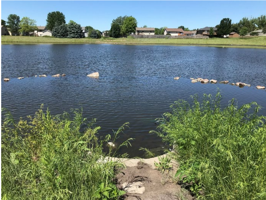
Figure 3.2 Stormwater site 5404 S Southwind Avenue
