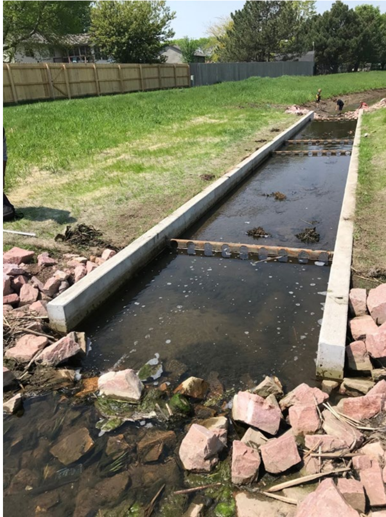
Figure 3.13 Overview of the stormwater filter structure
