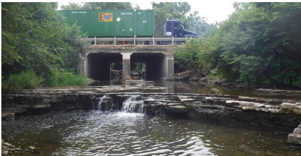
Figure 14. Photo. Example of multi-cell box culvert.
