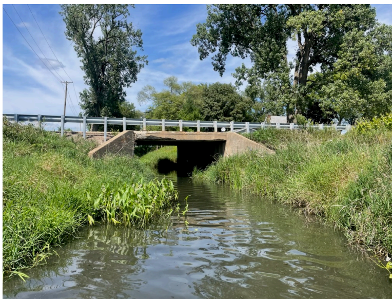
Figure 8. Photo. Example of a three-sided culvert or bridge culvert.
