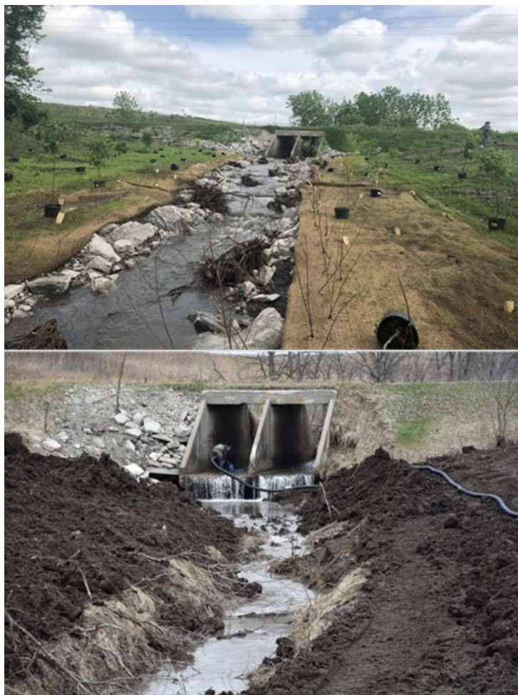
Figure 16. Photo. Example of grade control structure to assist with AOP.
