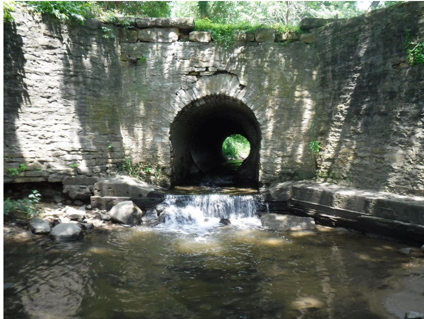
Figure 6. Photo. Example of an arch culvert.
