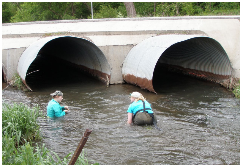
Figure 5. Photo. Example of a pipe arch culvert.
