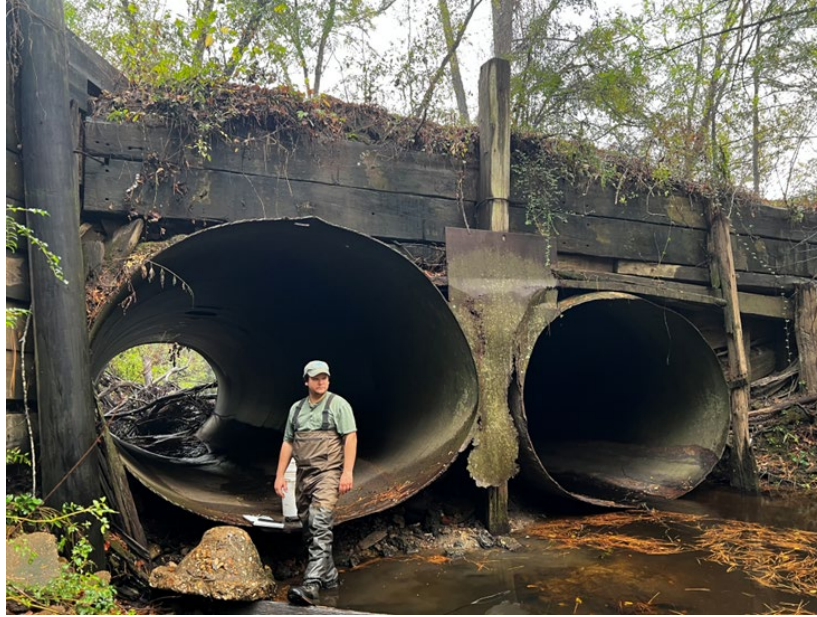
Figure 4. Photo. Example of a pipe culvert.
