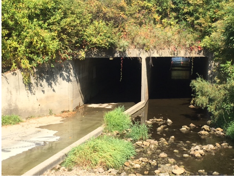
Figure 7. Photo. Example of a box culvert.
