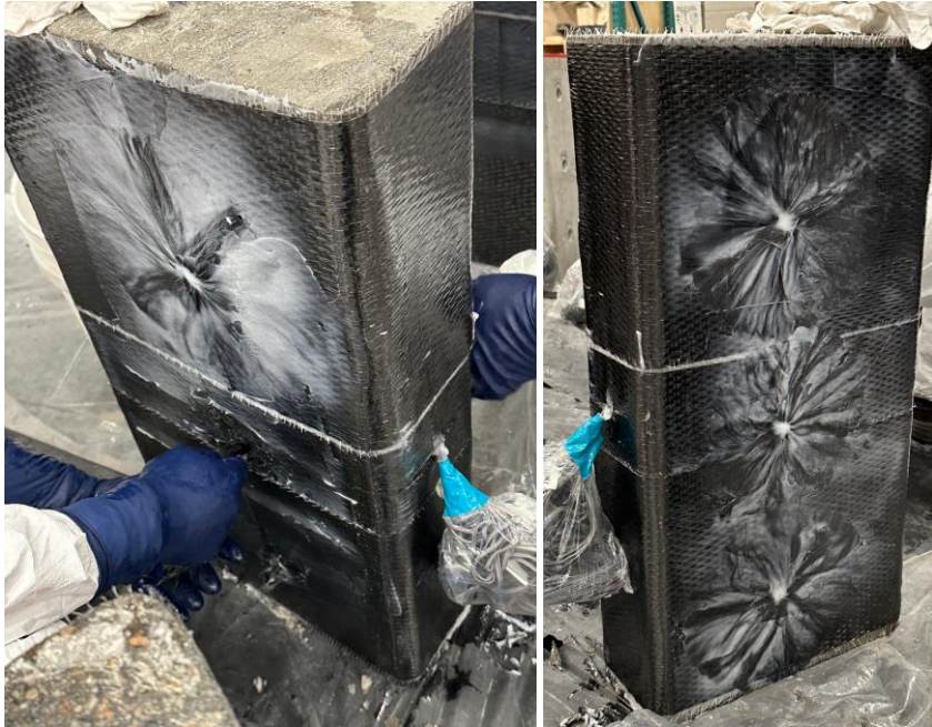
Figure 13 Inserting FRP anchors.
