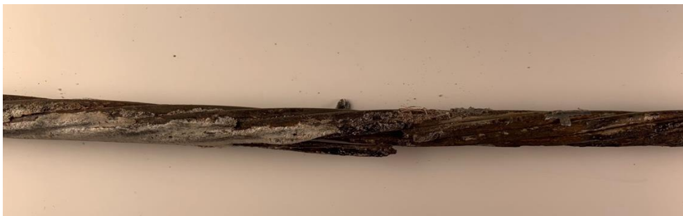
Figure 91. Strand Taken from Box Beam 4 after Testing
