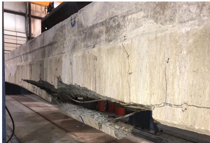
Figure 67. Box Beam 4 East Side after Testing
