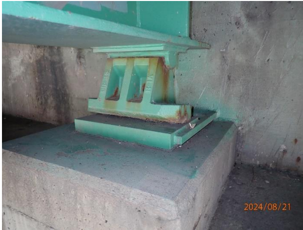
Figure 96. Rocker bearing on US 77 over Missouri River
