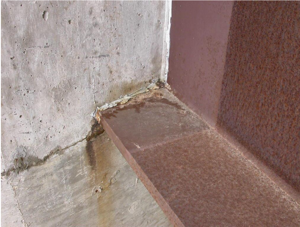
Figure 70. Photograph of rust products implying corrosion at an abutment belonging to No. 606750, dated May 6, 2015, from NBI inspection records.
