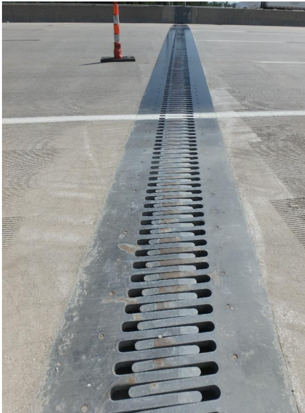
Figure 82. Finger joint on I-80 Westbound over Missouri River
