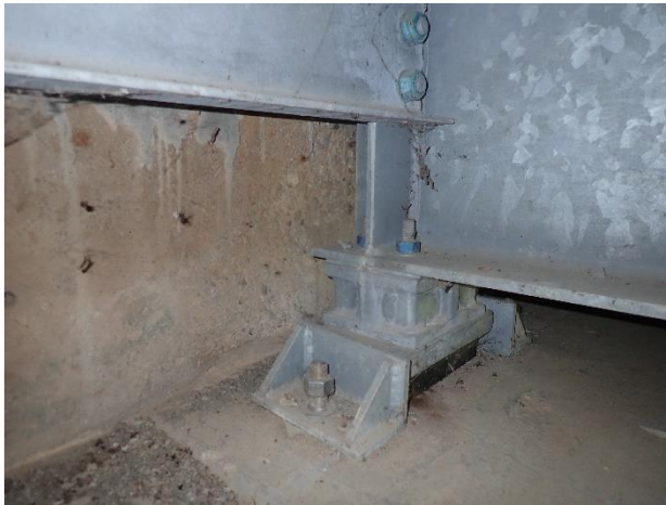
Figure 92. Steel-reinforced elastomeric bearing on Deerpath Road over East Skokie Ditch in Lake Forest, IL
