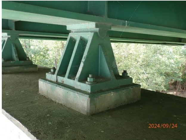
Figure 97. Fixed shoe on US 61 over Mississippi River
