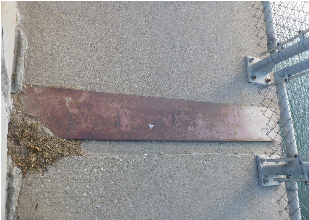
Figure 79. Sliding plate joint in sidewalk on Iowa 926 over the Des Moines River
