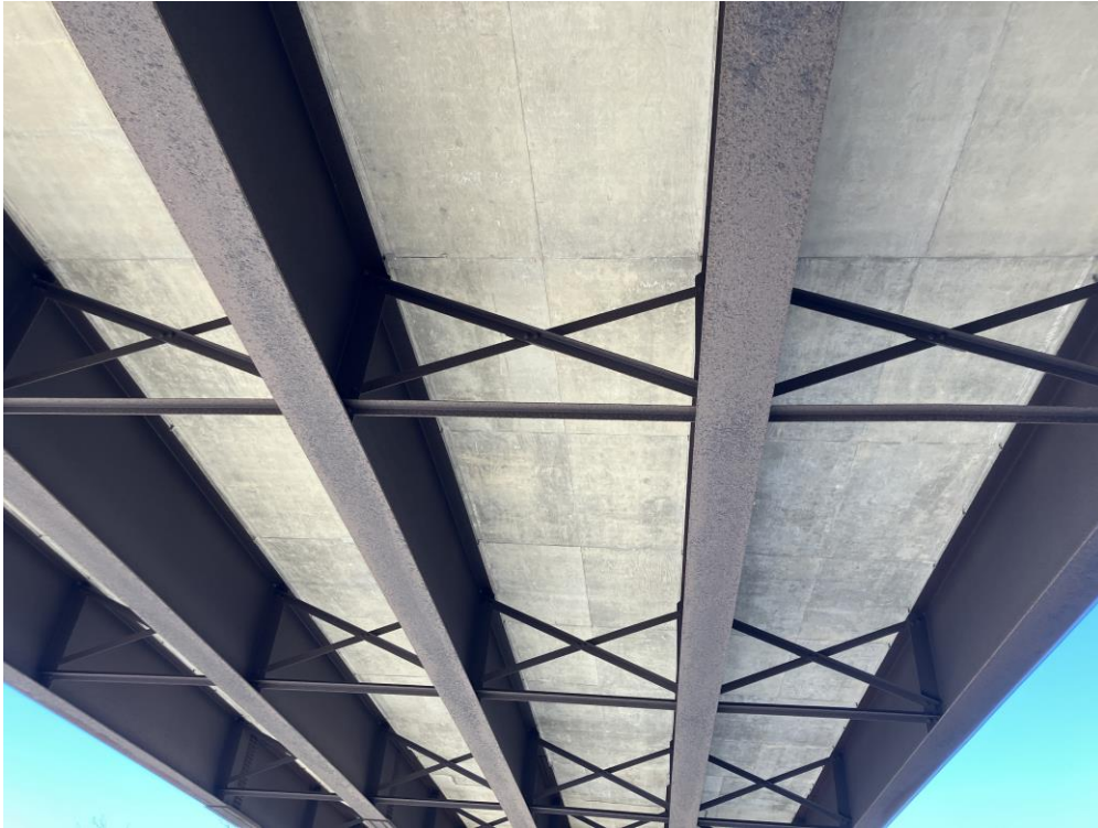
Figure 68. Photograph of the typical appearance of the floor system of No. 606750, dated December 12, 2023, from NBI inspection records.
