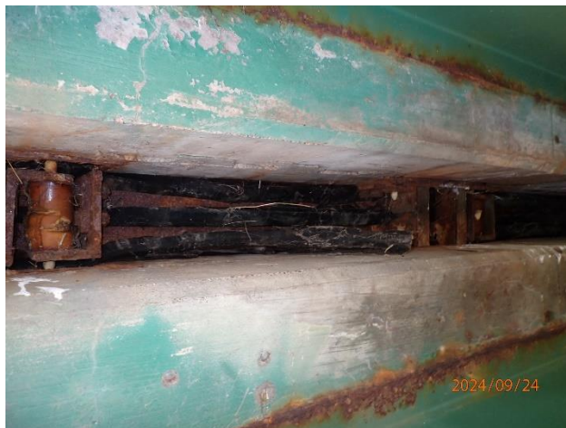
Figure 85. Underside of modular joint
