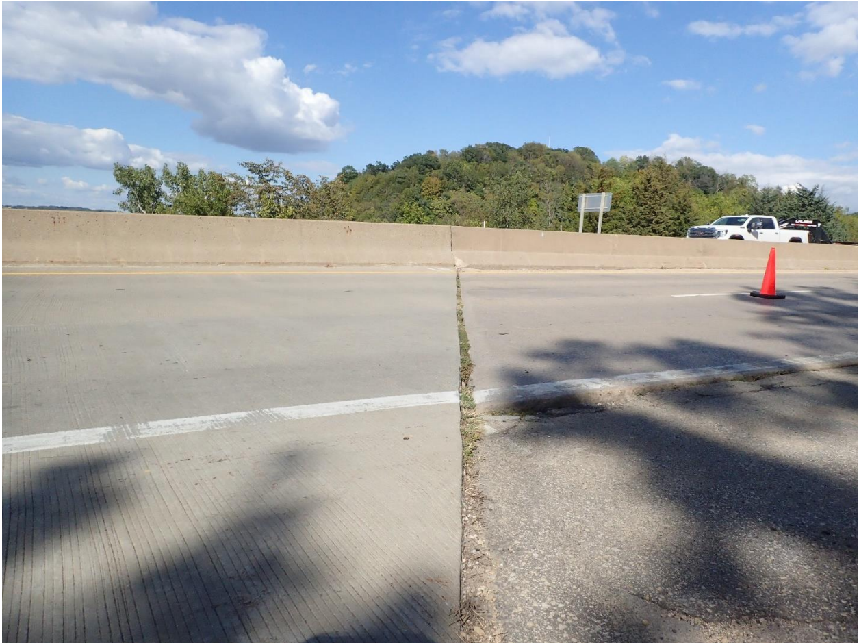
Figure 77. Pourable joint on US 62 over Mississippi River that has become an open joint
