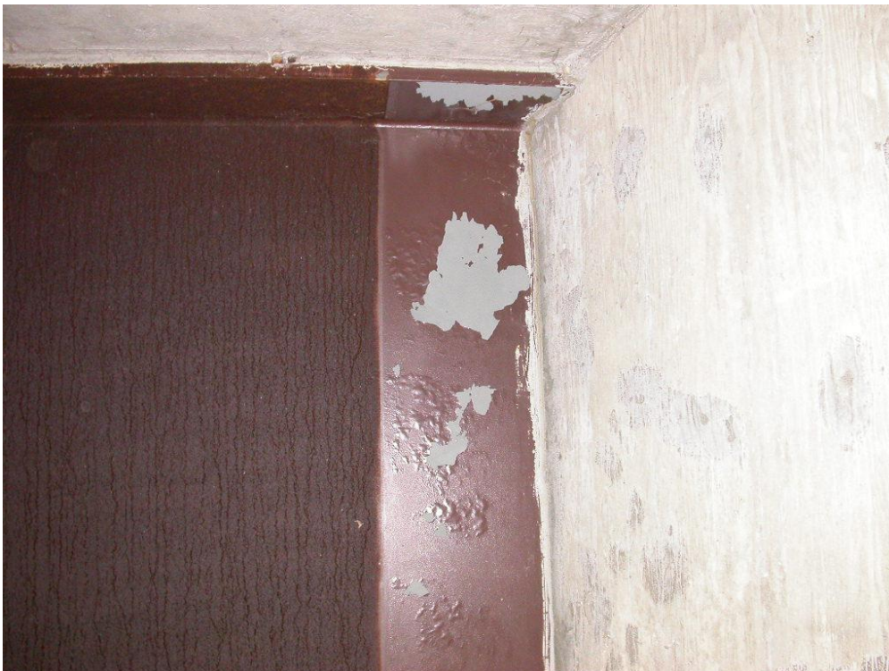
Figure 71. Photograph of peeling paint adjacent to an abutment belonging to No. 606750, dated May 6, 2015, from NBI inspection records.
