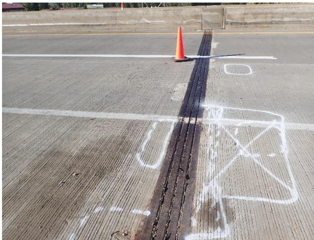
Figure 84. Modular joint on US 61 over Mississippi River
