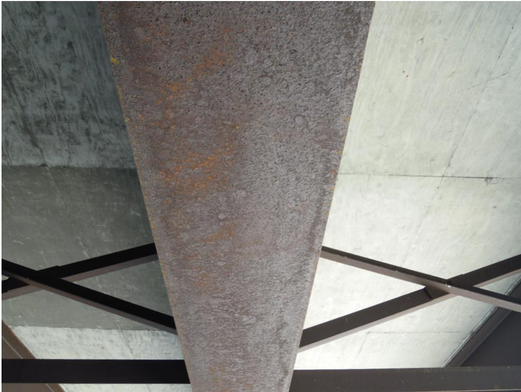
Figure 73. Photograph of typical “light flaking rust above roadways” on underside of a bottom flange of a girder belonging to No. 609280, dated September 29, 2010, from NBI inspection records.
