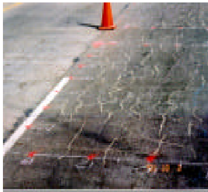
Fig. 2 – Bridge #2/Crack Pattern
