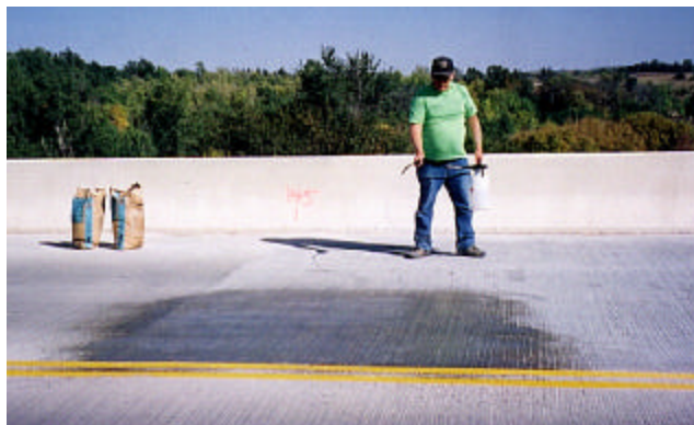
Figure 11 – Silanes & Epoxy Installation
