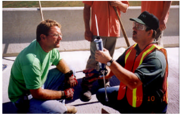
Figure 9 – MPU Cartridge Preparation
