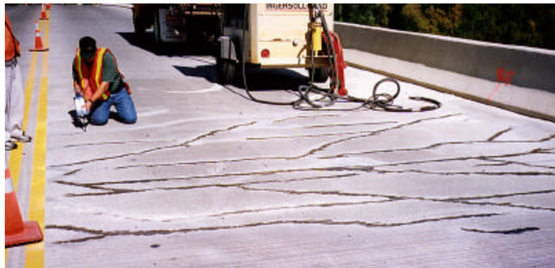
Figure 10 – MPU Installation
