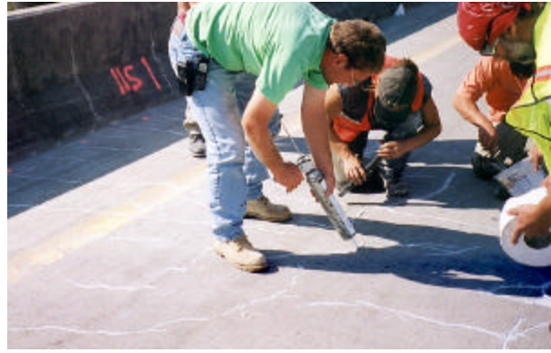
Figure 13 – Silicone Installation
