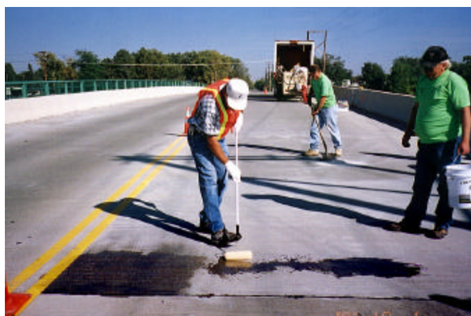
Figure 7 – MMA Roller Application
