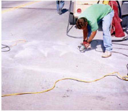
Figure 12 – Crack Preparation
