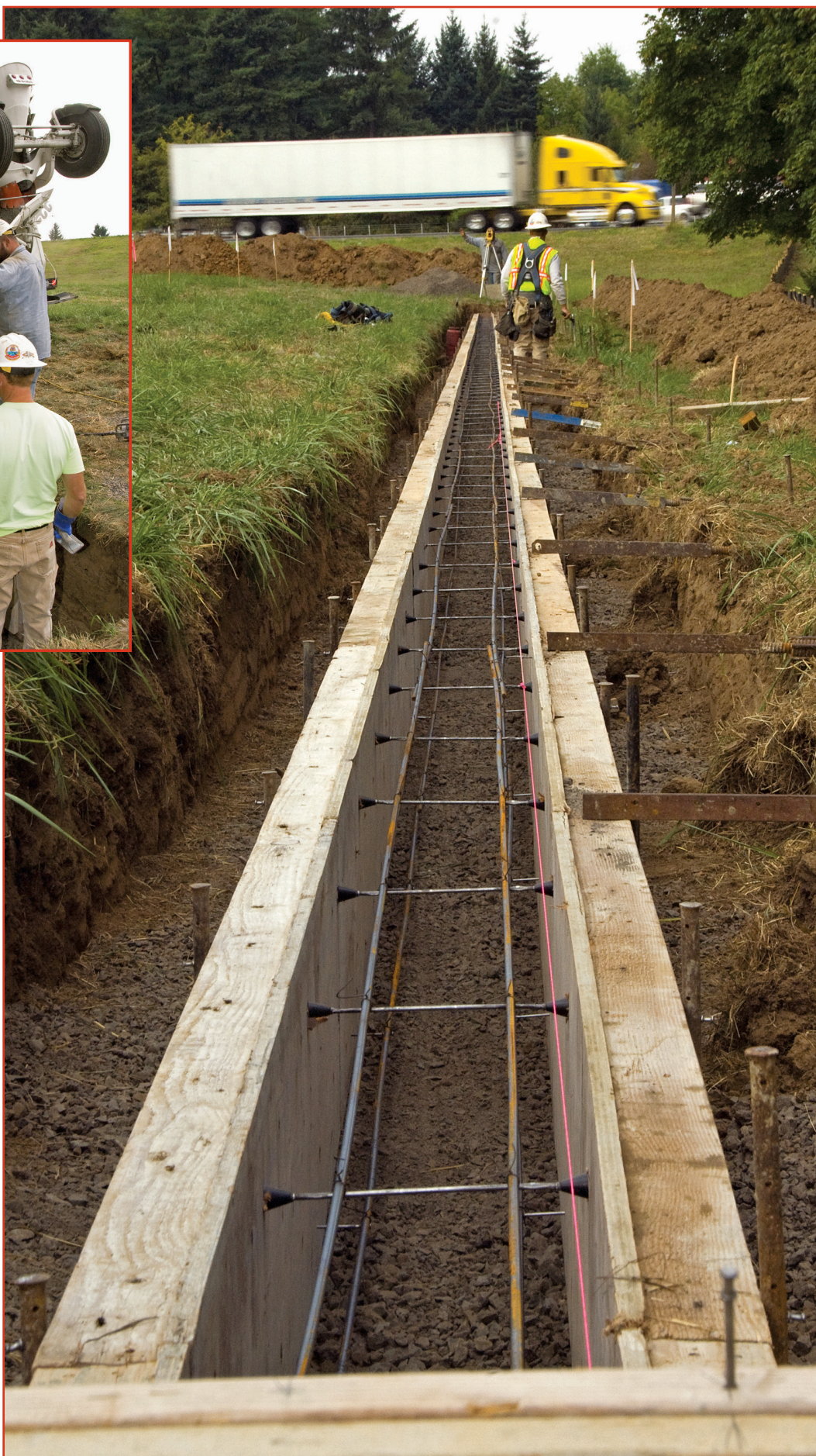
During the early stages of construction of the demonstration project, these workers were pouring concrete for the solar array's foundation.
