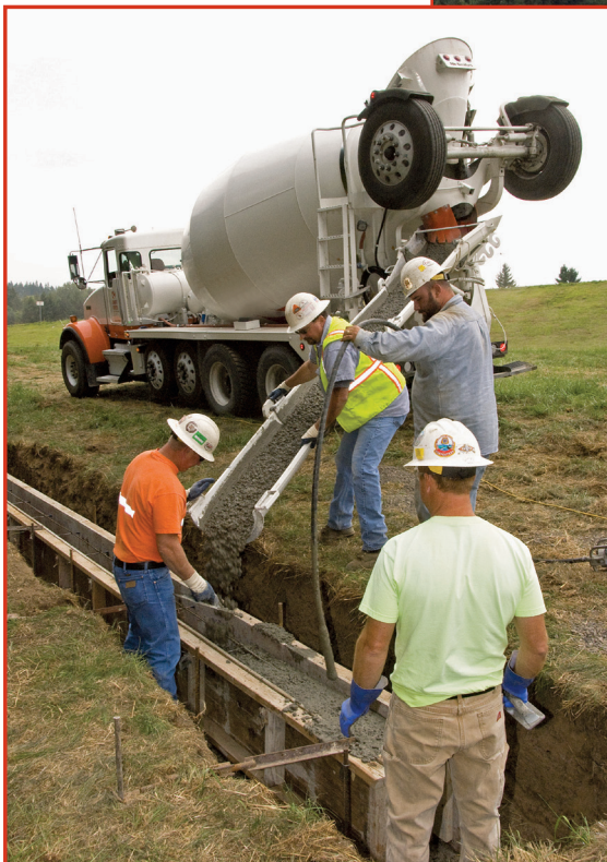
During the early stages of construction of the demonstration project, these workers were pouring concrete for the solar array's foundation.
