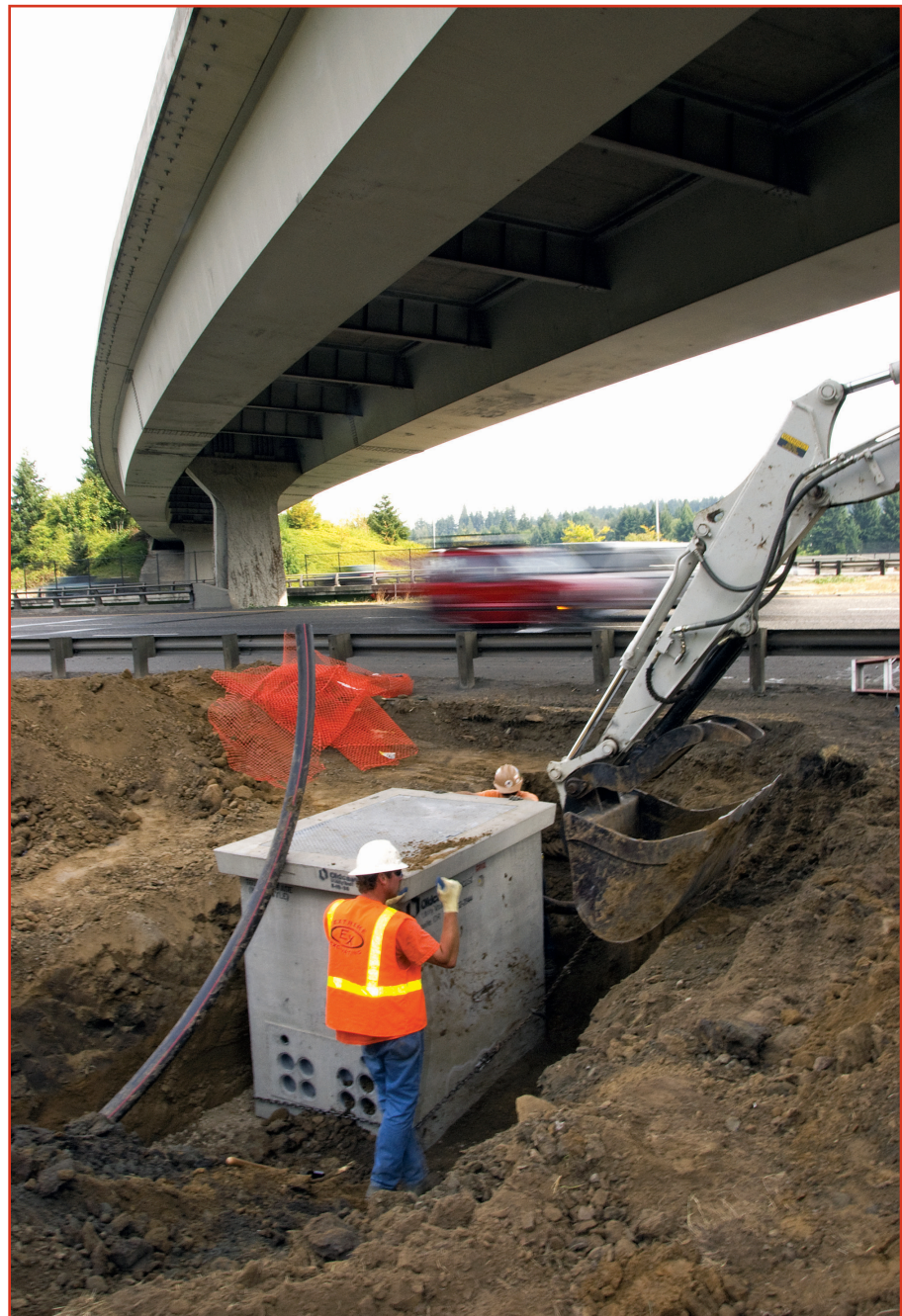
These workers are installing a power vault for the solar array.
