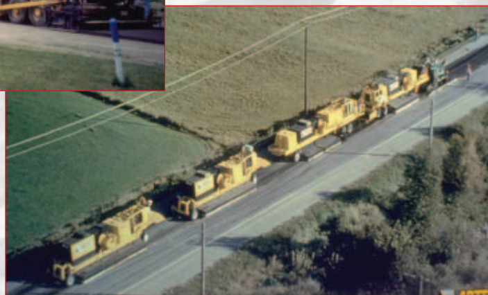
Hot in-place recycling equipment, shown in these two photos, is frequently referred to as a "train" and typically consists of heaters, heater-millers, a mixing machine, and pavers for HIR or a milling machine, crusher, and paver for CIR.
