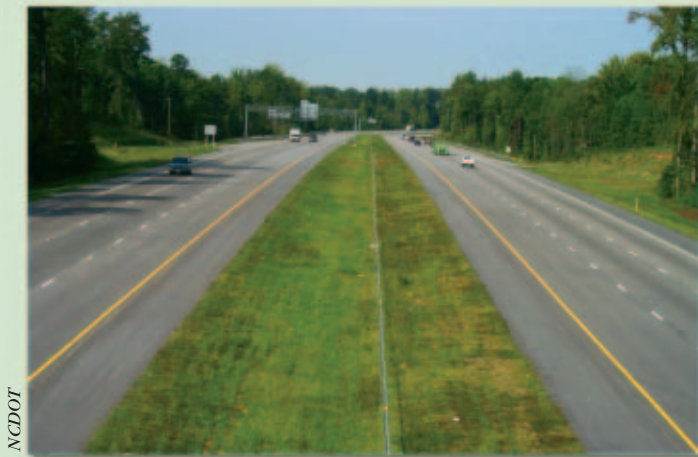
Another cable guardrail installation on Interstate 540 in Wake County, NC, showing an extremely narrow median.
