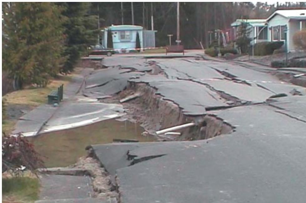
NHI's new course on the geotechnical aspects of pavement design will help transportation specialists avoid road collapses like this one caused by problems in the subgrade.
