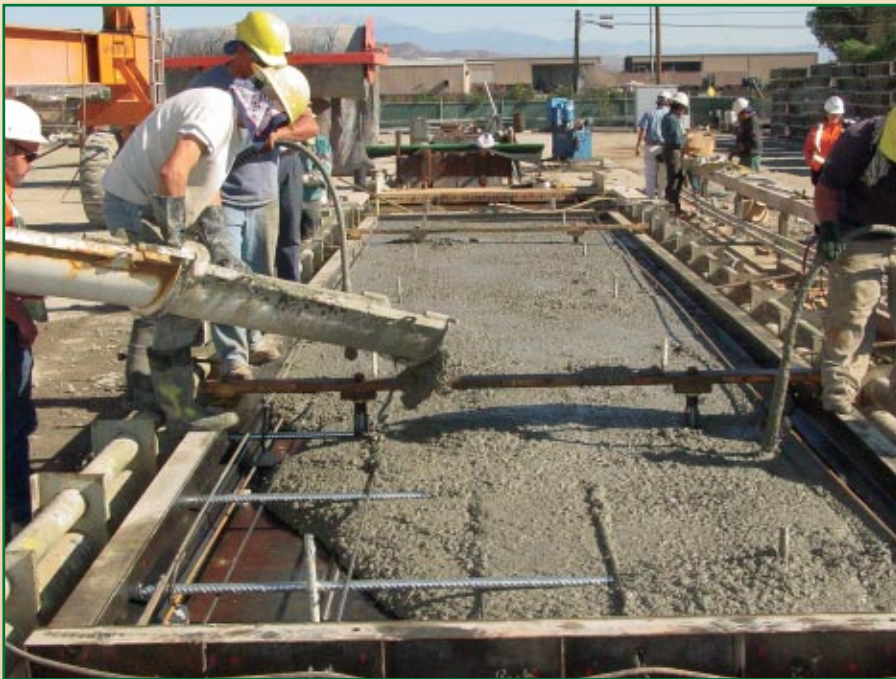
Workers place concrete for one of the panels used in the California demonstration project.
