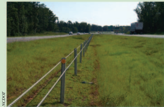
The North Carolina Department of Transportation installed this cable guardrail along Interstate 540 in Wake County, NC.
