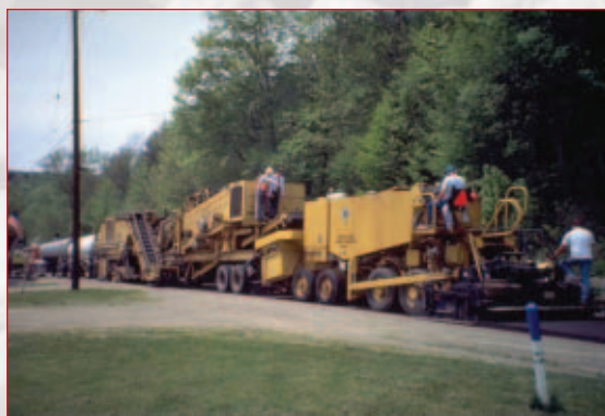
Hot in-place recycling equipment, shown in these two photos, is frequently referred to as a "train" and typically consists of heaters, heater-millers, a mixing machine, and pavers for HIR or a milling machine, crusher, and paver for CIR.
