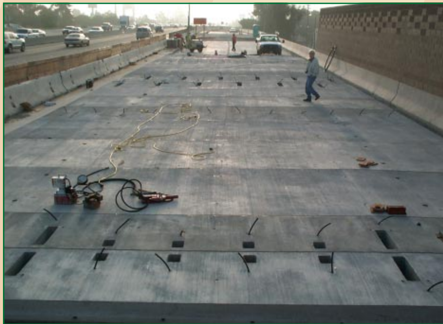
A worker surveys a 38-meter (124-foot) posttensioned section of precast pavement on the California jobsite.
