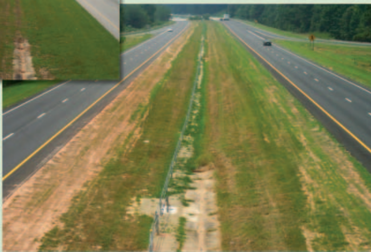
U.S. 64 in Franklin County, NC, before (inset) and after installation of a cable barrier. The guardrail was installed as part of a repaving and shoulder rehabilitation project.
