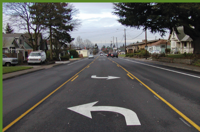
(Left) Fourth Plain Boulevard in Vancouver, WA, before road diet conversion. (Right) Fourth Plain Boulevard after conversion. Photos: City of Vancouver.
