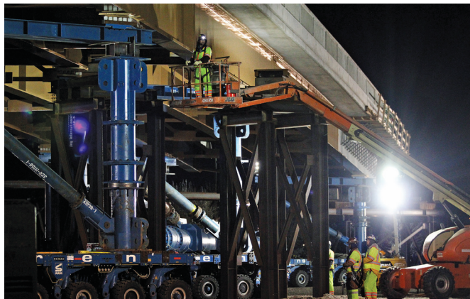
UDOT's I-15 Corridor Expansion crew members prepare to move the Sam White Bridge, shown here lifted on the hydraulic self-propelled modular transporters.
