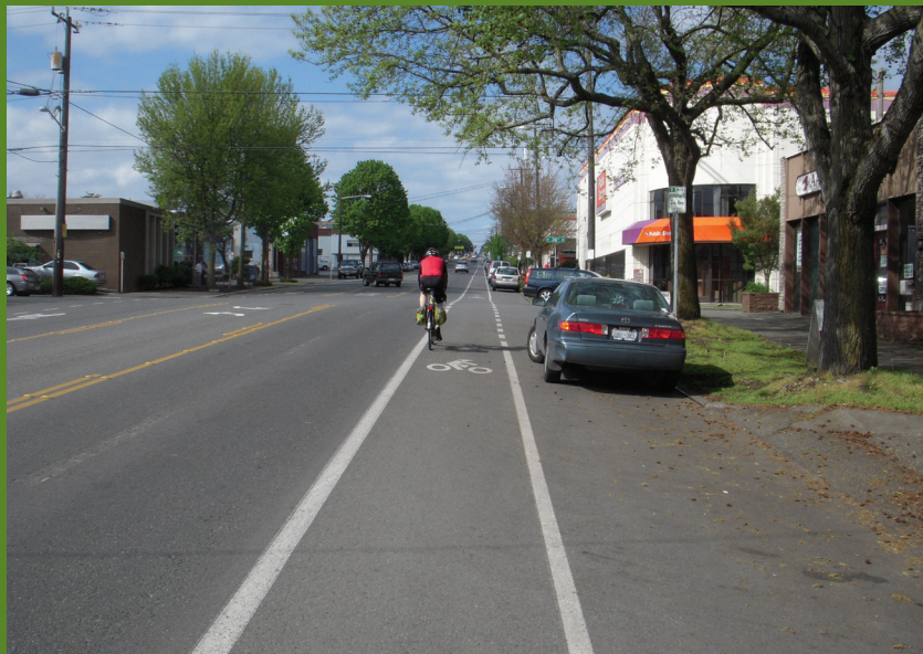
(Top) Stone Way North in Seattle, WA, looking north at N 36 th Street before the road diet conversion. The roadway surface was in poor condition, there were no bicycle facilities, and there were several uncontrolled marked crosswalks where pedestrians had to navigate across four lanes of traffic. (Bottom) Stone Way North looking north from the same vantage point after the conversion. The roadway was resurfaced, one travel lane in each direction was provided, along with a two-way left-turn lane. A dedicated bicycle lane was added uphill with shared lane markings downhill. Pedestrian crossings were upgraded to include high-visibility fluorescent-green signage. Photos: SDOT.
