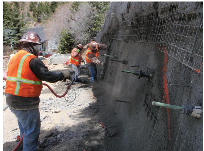
Workers are constructing the facing for a permanent soil nail wall on a project in Guanella Pass near Georgetown, CO.
