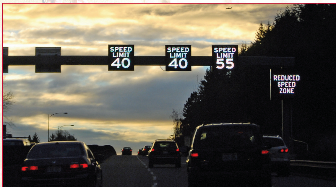
These overhead electronic signs on SR-520 in Bellevue, WA, display different speed limits for each lane.
