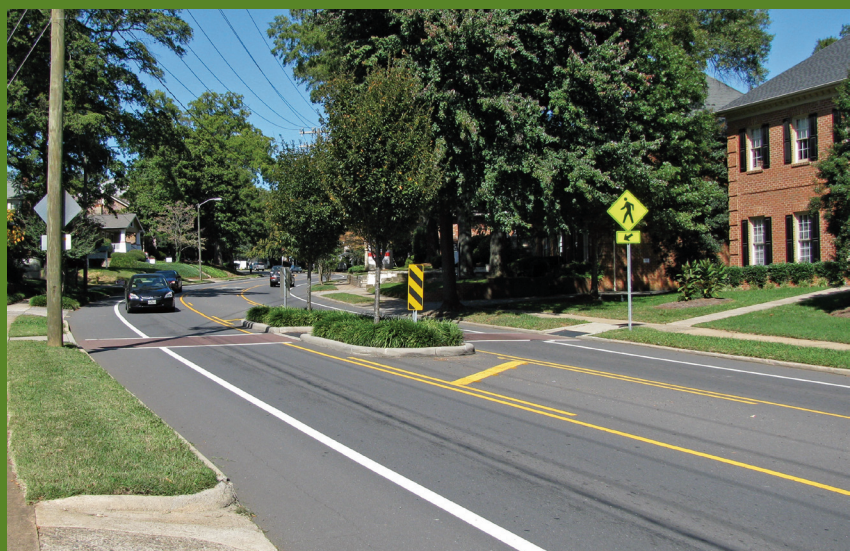
(Top) This "during construction" photograph shows a four-lane road in a neighborhood in Charlotte, NC. (Bottom) As shown in this "after" photo of the same location, reclaiming road space by turning the four-lane road into two lanes plus bicycle lanes created room for a pedestrian refuge island. Photos: Dan Gallagher.
