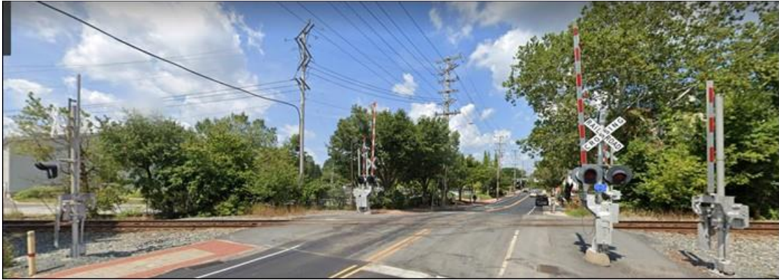
Figure 1: Typical Highway-Rail Grade Crossing with Gates
