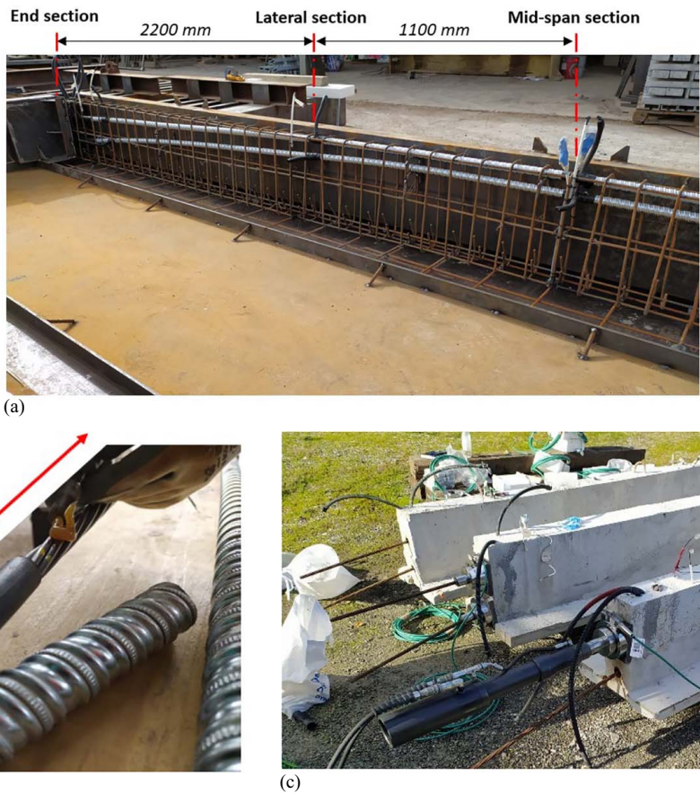
Fig. 3. (a) Side view of the upside-down girder in the steel formwork prior to casting; (b) polyurethane jacketing of 1 m of tendon for partially bonded (PB) configuration; and (c) hydraulic jack and load cells during prestressing.
