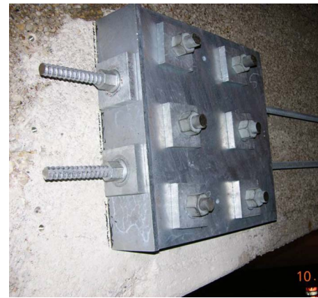
Fig. 13. Transverse pretensioned rods (six rods per bracket)
