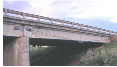
Fig. 3. External posttensioning using draped profile cables
