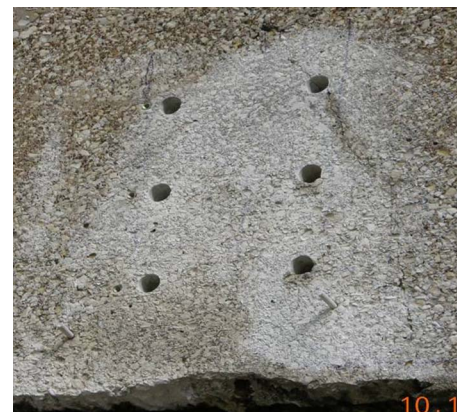
Fig. 15. Six holes drilled through the exterior girder in the transverse direction
