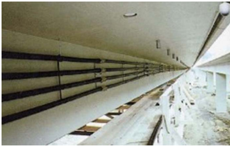
Fig. 1. External posttensioning using straight profile cables
