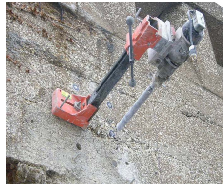
Fig. 14. Drilling holes through the exterior girder in the transverse direction
