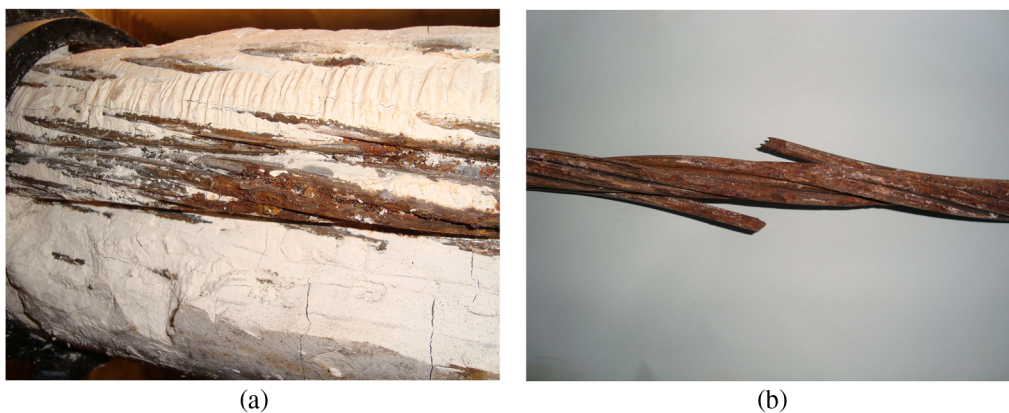
Fig. 1. Examples of (a) whitish segregated grout in the external posttensioning tendons; (b) severe corrosion attacks on a strand that was in contact with this grout
