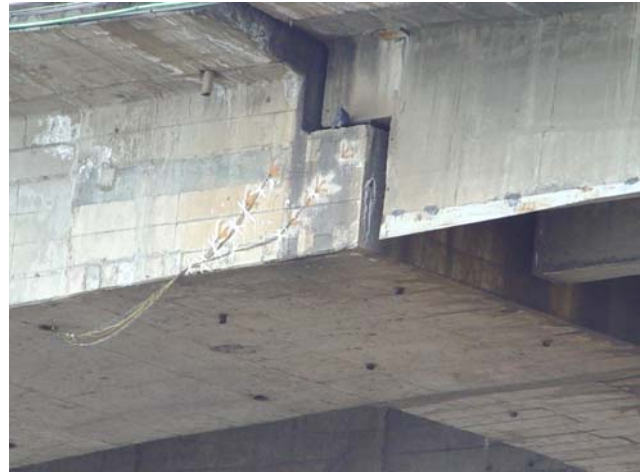
Figure-6. Damage of corbel
