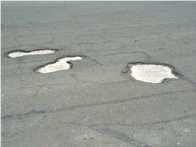
Figure-3. Damage of deck pavement.
