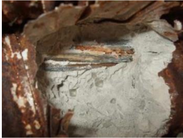
ID-4.7. View of the non-Portland cement grout for the bonding of tendons and advanced corrosion of both duct and strands (Anania et al, 2018).
