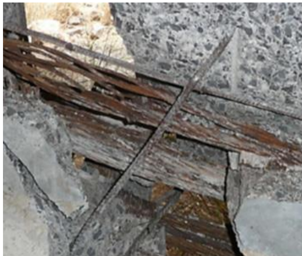
ID-4.3. Tendons in the bridge after collapse (Anania et al, 2018).
