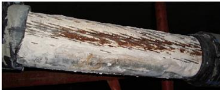
ID-18.2. Example of whitish segregated grout embedding corroding strands (Bertolini and Carsana, 2011).
