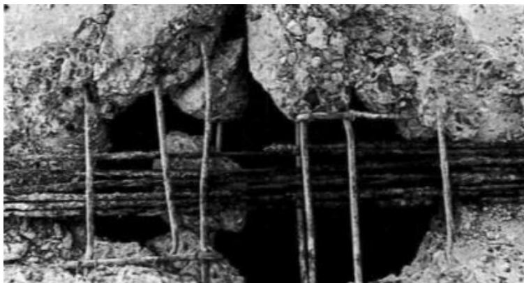
ID-1.6. Transverse tendon crossing a longitudinal joint: duct poorly grouted and corrosion on wires within segments (Woodward and Williams, 1988).
