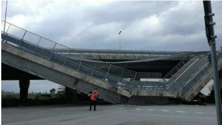
ID-5.1. Collapse mechanism of the bridge
