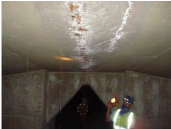
ID-13.2. Presence of efflorescence, delamination, and spall observed on post-tensioned box girders (Venugopalan, 2008).
