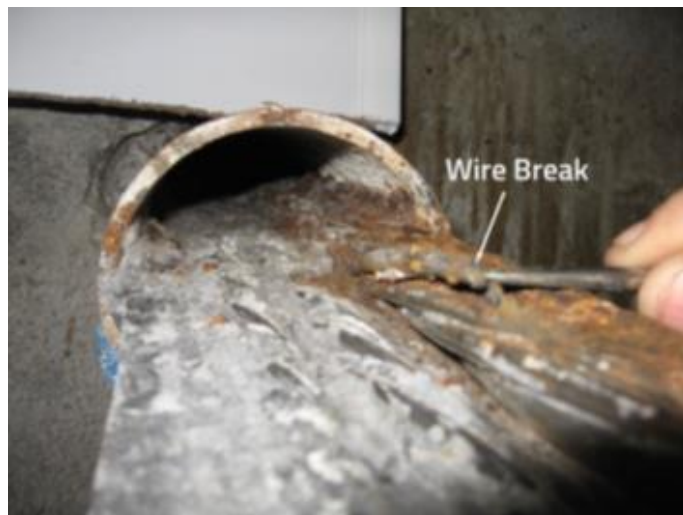
ID-15.4. Corrosion of strands and wire breaks identified in other external PT tendons (Ahern et al, 2018).
