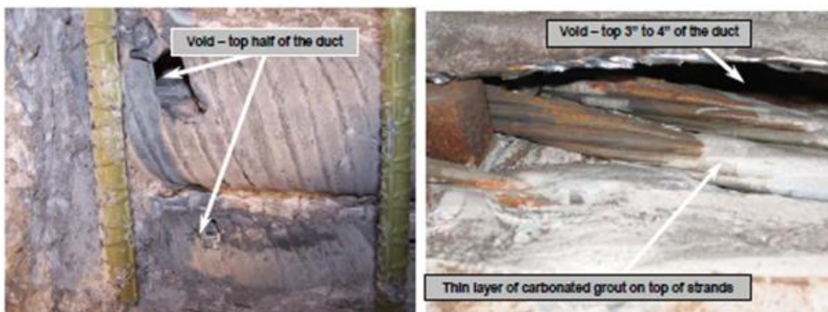
Figure 13.3. Voids (with a thin layer of chalky material) at different sections of the tendon. (Venugopalan, 2008).
