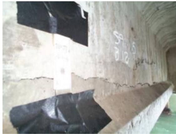
ID-3.2. Typical longitudinal web cracking along a beam (Papè and Melchers, 2011).
