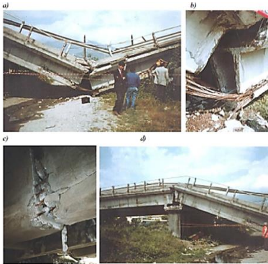
ID-2.3. S. Stefano Viaduct: a) collapse of the viaduct; b) slippage of cables; c) opening of joints; and d) rotation of the deck (Colajanni et al, 2016).
