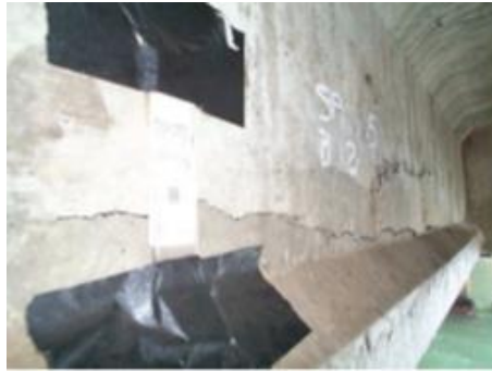
Figure 3.1.21. Typical longitudinal web cracking along a beam in Sorell Bridge (ID-3) (Papè and Melchers, 2011).
