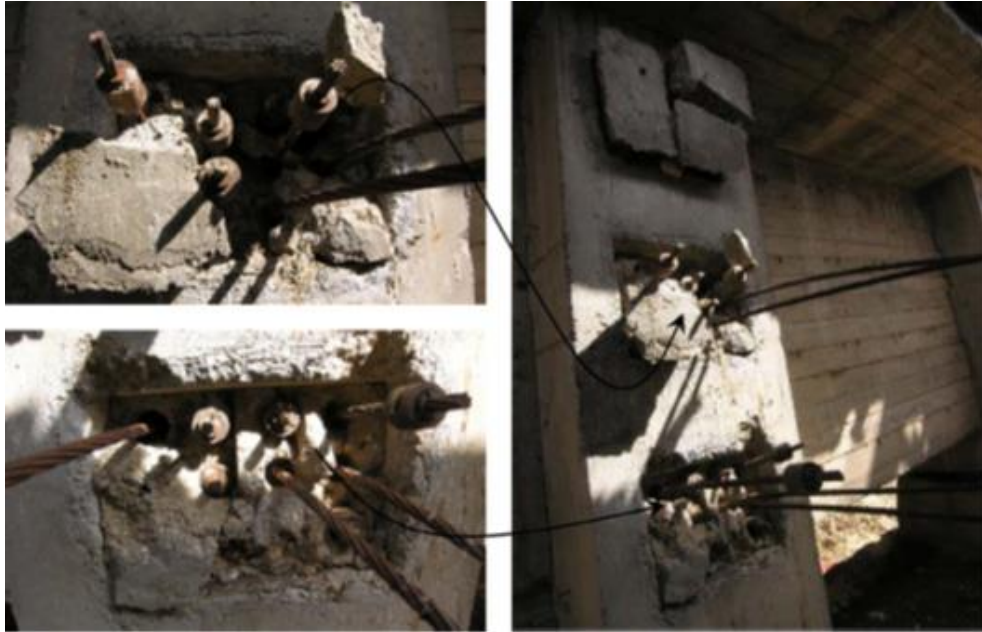
ID-4.4. Expulsion of the ducts head anchorages. Global view of the expulsion at the head of the girder beam (Anania et al, 2018).
