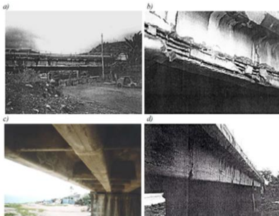
ID-2.2. S. Stefano Viaduct: a) beam shore side; b) details of corrosion phenomena on the shore side beam; c) bottom view of the deck; and d) damage on the beam mount side beam (Colajanni et al, 2016).
