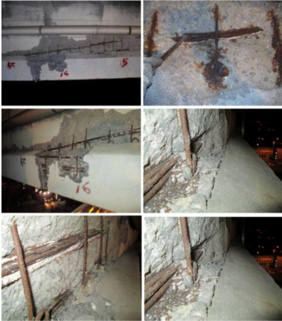
ID-6.7. View of cables toward the support in 2011 (top) and 2013 (middle). Zoom of the cables in 2013 (bottom) where corrosion and partial pitting can be appreciated (Nuti et al, 2020).
