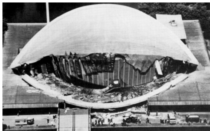
ID-19.5. View from the South on the collapsed roof overhang in 1980 (Helmerich and Zunkel, 2014).
