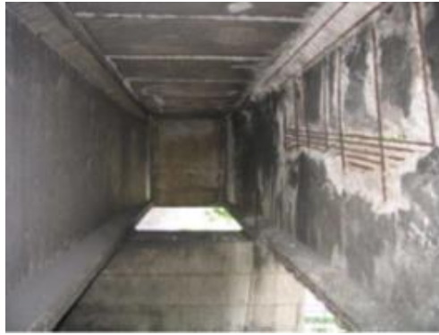
Figure 3.1.19. Annone Overpass (ID-21). Damage observed on internal surfaces of the prefabricated beams in 2006 (Di Prisco et al, 2018).
