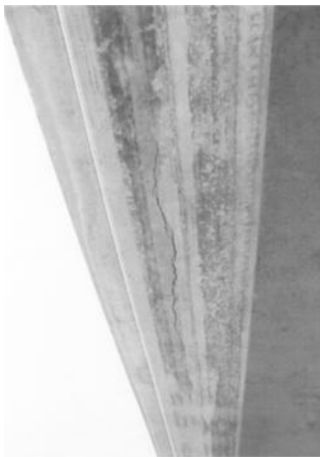
ID-9.5. Longitudinal crack in double-T beams stem directly under the grout plug location (Poston and West, 2005).
