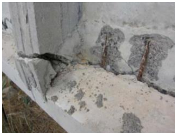
ID-4.9. Detailed view of vertical mild reinforcement expelled by the rotation of the lower flange (Anania et al, 2018).
