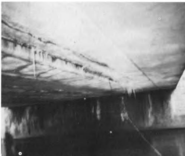
ID-31.6. Ruptured strand hanging down into river (Murray and Frantz, 1992).
