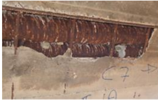
Figure 4.2.1.1. No gap among the tendons in Petrulla Viaduct (ID-4) (Anania et al, 2018).
