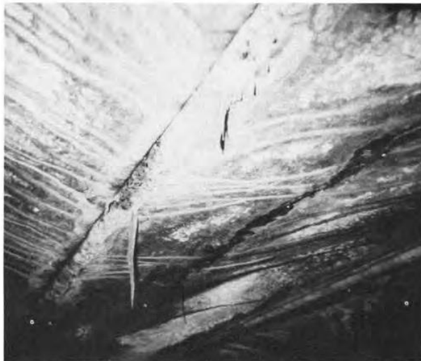
ID-31.5. Stains on beams (Murray and Frantz, 1992).
