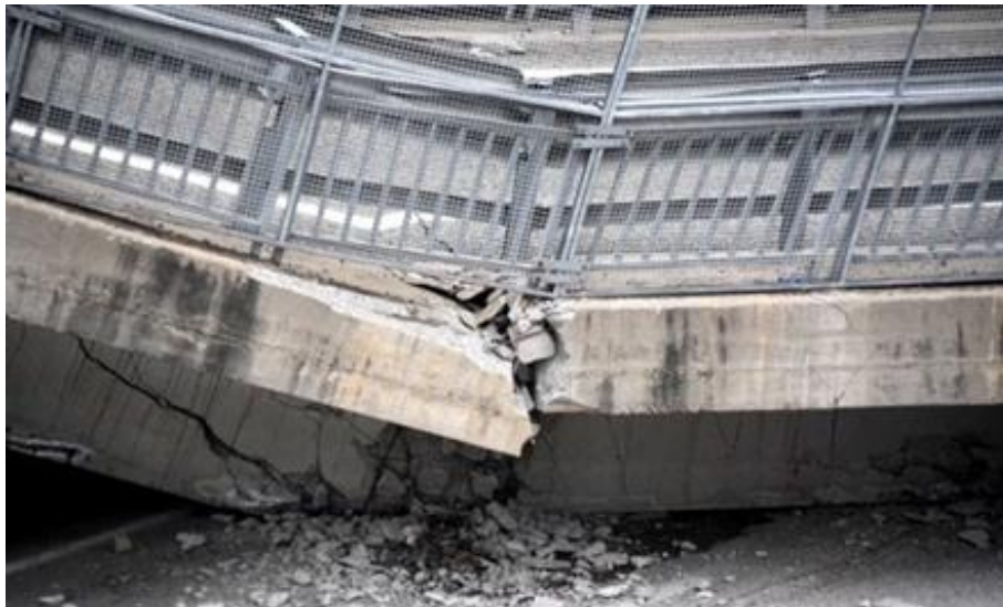
ID-5.2. Bridge beam: mid span fracture
