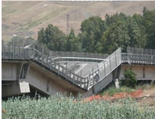
ID-4.1. Collapse mechanism of the bridge (Anania et al, 2018).
