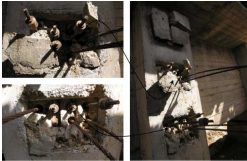
Figure 3.1.7. Petrulla Viaduct (ID-4). Expulsion of the anchorages. Global view of the expulsion at the end of the beam (Anania et al, 2018).
