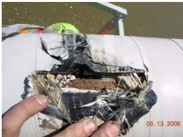
ID-10.2. Corrosion of wires at PE split (Mehrabi, 2009).
