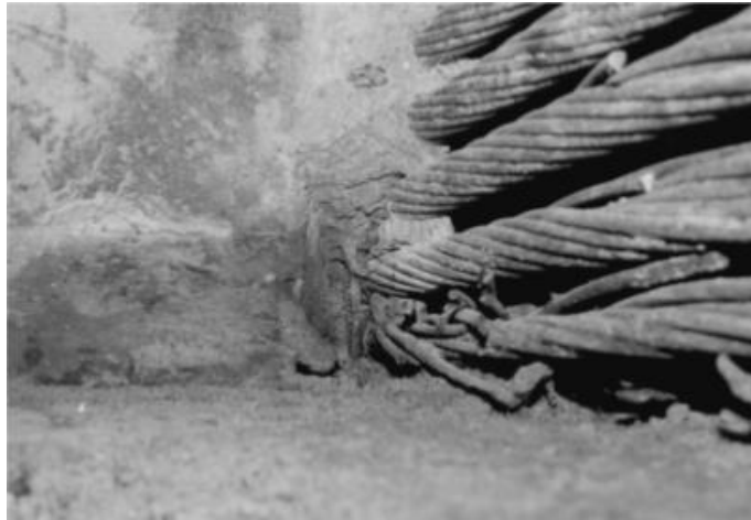
ID-28.1. Corrosion of external tendons that had been encased in concrete (Tilly, 2002).
