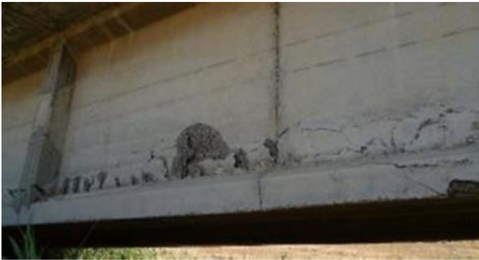
ID-4.8. Cracking in the other bridge spans (Anania et al, 2018).
