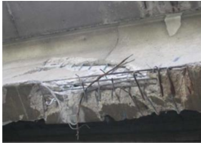
ID-21.5. Lateral impacts occurred in 2006 due to trucks circulating on SS.36 towards Lecco: particular of the damaged zone (Di Prisco et al, 2018).
