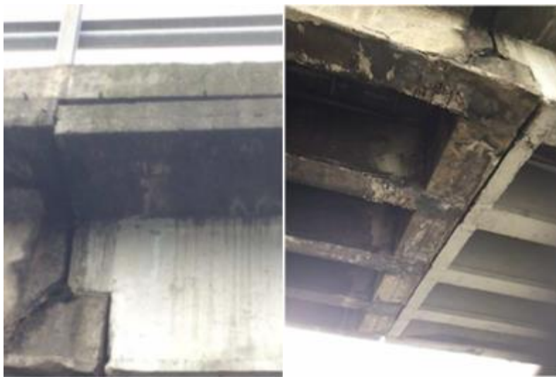
Figure 3.1.20. Annone Overpass (ID-21). Critical Gerber joint view before the collapse (Di Prisco et al, 2018).
