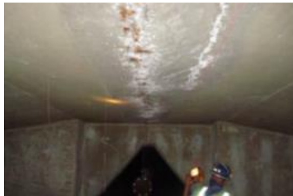
Figure 3.1.23. Bridge in the Midwest, USA (ID-13). Presence of efflorescence, delamination, and spalling observed on post-tensioned box girders (Venugopalan, 2008).
