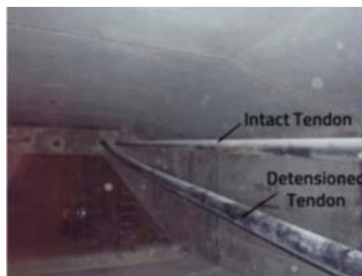
Figure 3.3.7. Ringling Causeway Bridge (ID-15). Detensioned tendon discovered in July 2011 (Ahern et al, 2018).
