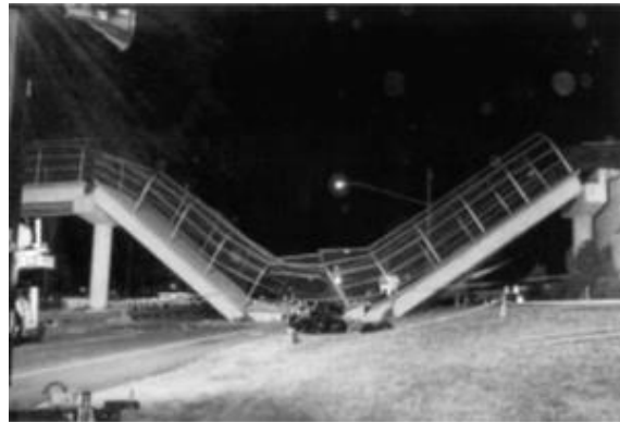
Figure 3.1.11. Collapsed span of Lowe’s Motor Speedway (ID-9) (Poston and West, 2005).
