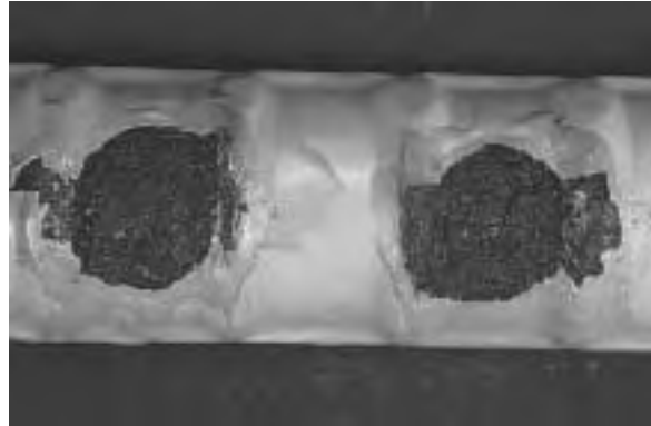
(b) Corrosion of steel surface beneath patched areas.
