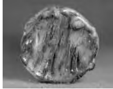
(b) Corrosion of patched end (torch-cut).
