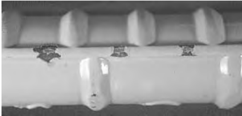
(a) Coating damage on longitudinal rib.
