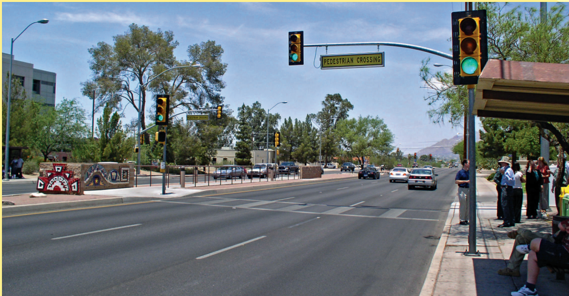
Shown here is a PEDESTRIAN Light Control Activation (PELICAN) crossing—a two-stage pedestrian signal-actuated crossing—at the University of Arizona Medical Center in Tucson, AZ.
