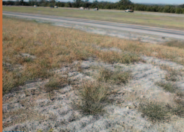
These soil erosion blankets along Spur 208 in the Dallas area failed to establish grass.
