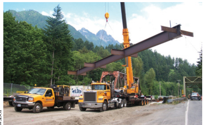
A crane hoists a girder for the temporary bridge that will detour motorists around construction of the new Barclay Bridge on U.S. 2, east of Everett, WS. The old bridge is shown in the lower right corner.
