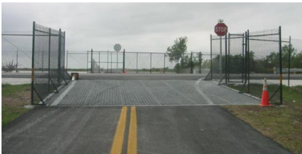
This completed deer guard (with fencing) is located at a side road that intersects U.S. 1 in the Florida Keys.
