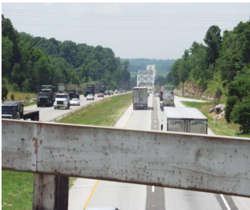
I-70 in Missouri, shown from an overpass, is one of the Nation's oldest interstates, built between 1956 and 1965. It is characterized by aging pavement, a narrow median, and narrow shoulders.
