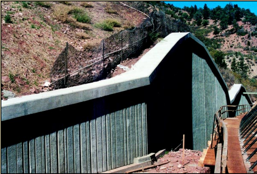
A precast architectural panel covers a soil-nail wall.
