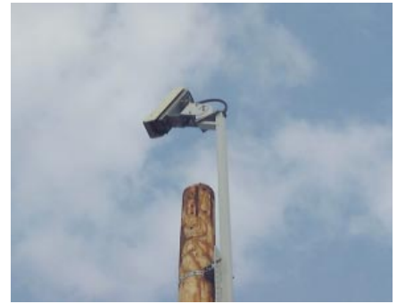
A video camera mounted on a temporary wood pole shows one way to install AIRS.
