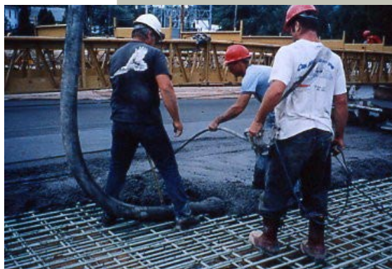
Workers place high-performance concrete (HPC) on a bridge deck in New Hampshire. The Resource Center recently held an Internet conference on HPC. Photo: HPC Bridge Views, a publication sponsored by FHWA and the National Concrete Bridge Council.
