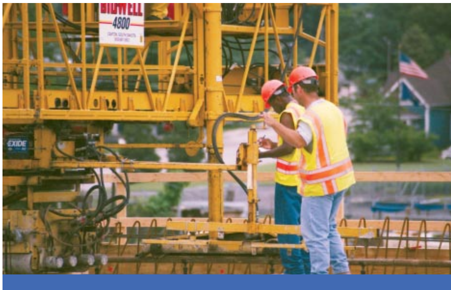
Workers prepare to place bridge deck overlays.
