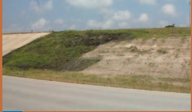
(After) TxDOT smoothed the slope and applied erosion control compost. This photo shows the same slope 2 weeks after compost was applied.
