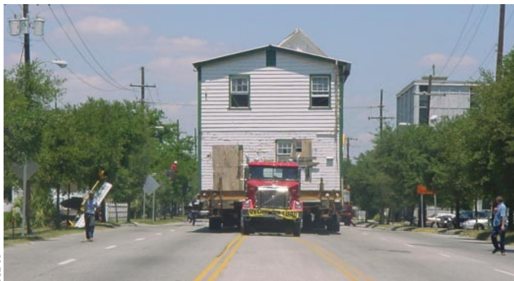
This house in Charleston, SC, was scheduled for demolition, but here it is being moved for donation to the city of Charleston to use for affordable housing.
