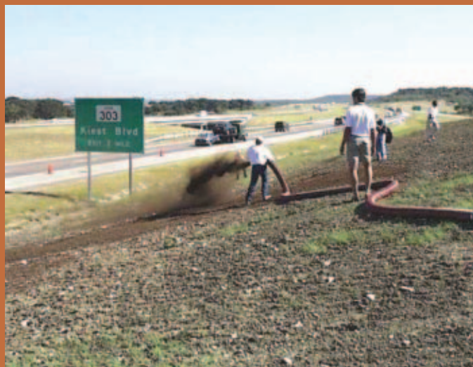
Composted dairy manure is applied to Spur 208 in Dallas.
