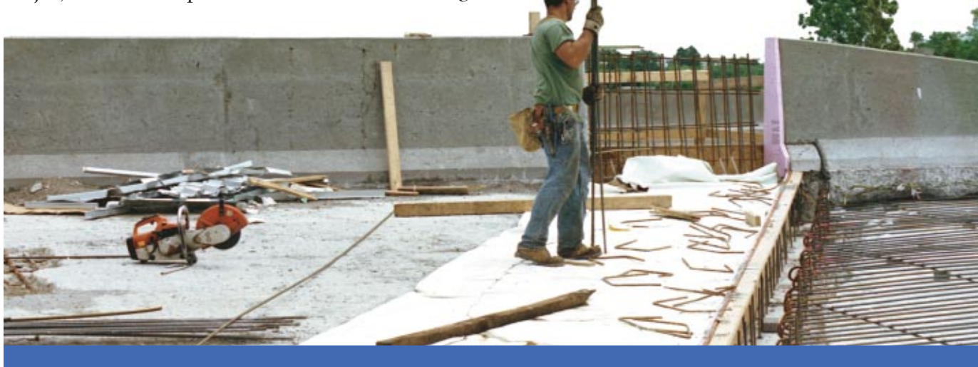
Another worker gathers rebar for an approach slab for a bridge deck.
