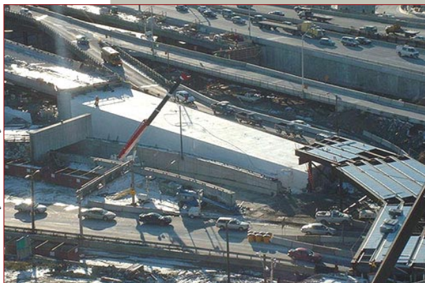
The use of expanded polystyrene (EPS) geofoam as a lightweight fill material for highway embankments on the Boston's Central Artery/Tunnel Project originated at the suggestion of FHWA.
