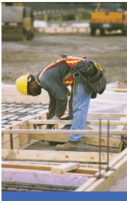
A worker sets up a form for concrete placement on a bridge deck approach.
