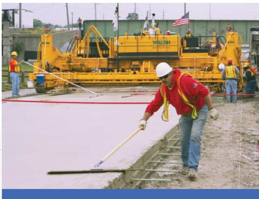
A construction worker smoothes the concrete for the new highway during the Hyperfix 65/70 project.
