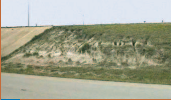
(Before) Erosion along State Highway 47 in College Station, TX, threatens this riprap slope. Left alone, the erosion would be expensive to repair.
