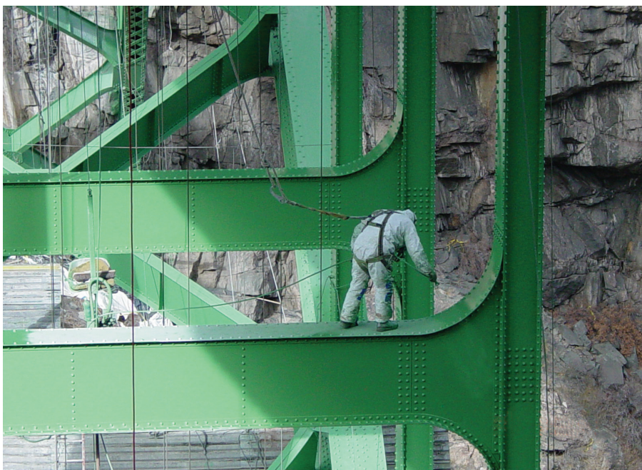
A worker wearing a safety harness and protective clothing is spraying a new coat of paint on a bridge girder.
