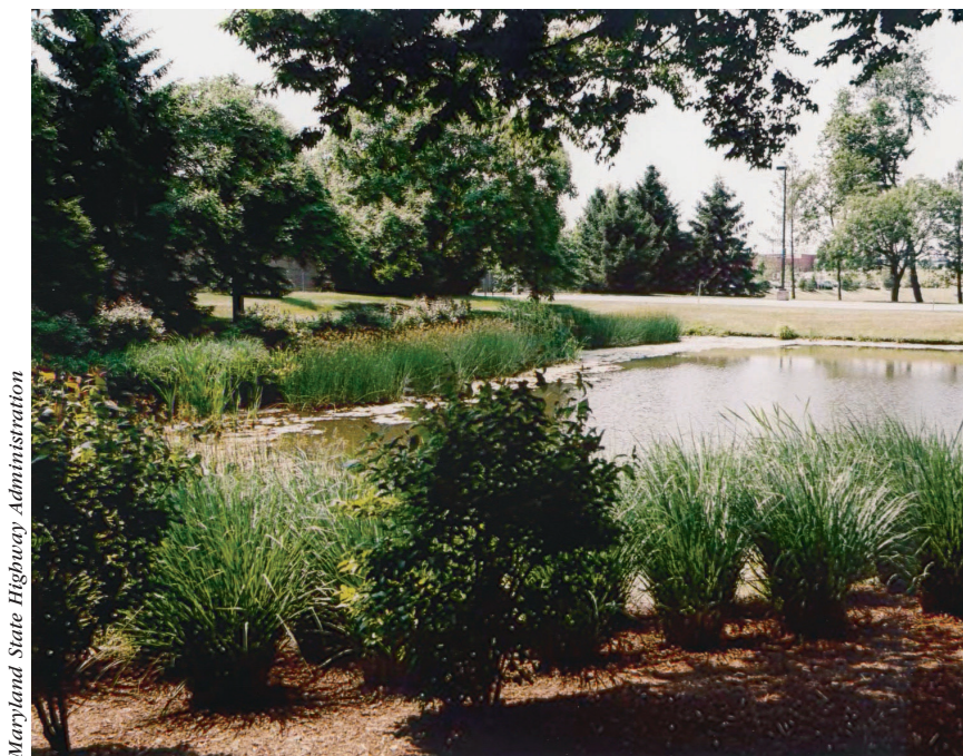
On this highway project, the Maryland State Highway Administration used a comprehensive maintenance program to locate, inspect, evaluate, remediate, and enhance all of the stormwater management facilities to improve water quality and protect sensitive wetlands and water resources. The retention pond is surrounded by a vegetated fringe that promotes ecological diversity, enhances water quality, and fits harmoniously with the local environment.
