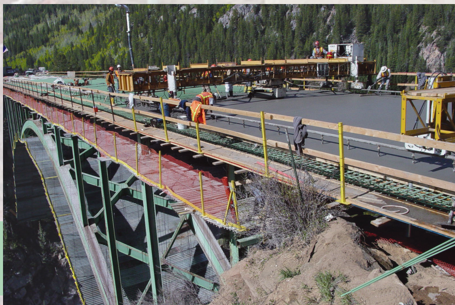
Workers use a screed and finishing machine to smooth the concrete applied during the second deck pour on the north end of the bridge.
