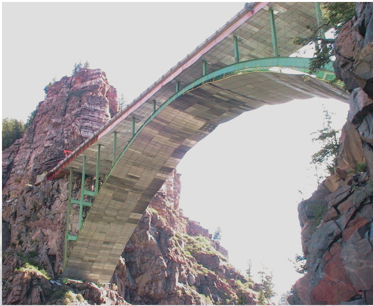
Scaffolding installed under the bridge deck (above) provides a safe and efficient platform for the workers and inspectors. A view of the bridge from below (left) shows the scaffolding in place beneath the arch, where it helps protect the county road and river from falling objects.
