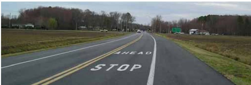
Figure 1. Example of a Rural STOP AHEAD Installation.
