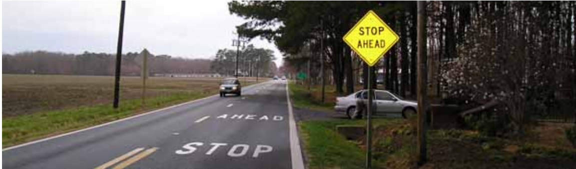
Figure 2. STOP AHEAD Pavement Marking with Warning Sign.
