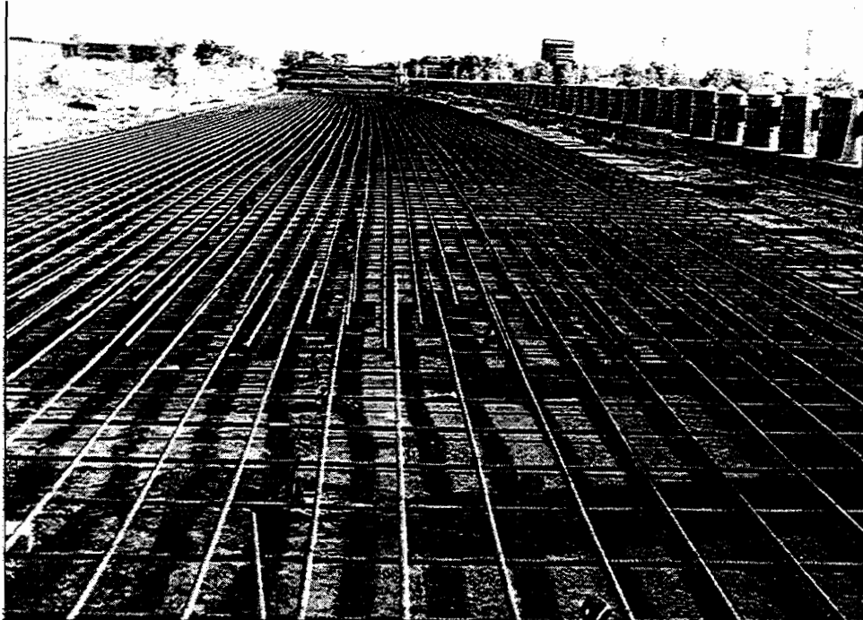
Figure 2.2 Typical steel lap technique between sections with different steel design
