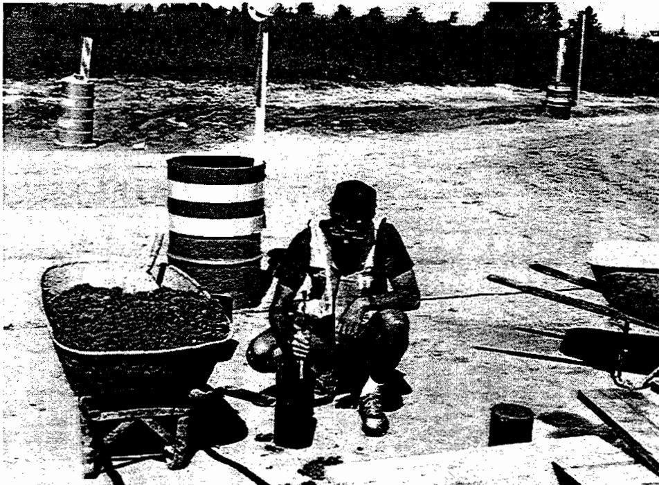
Figure 2.13 Cylinders being cast in the field
