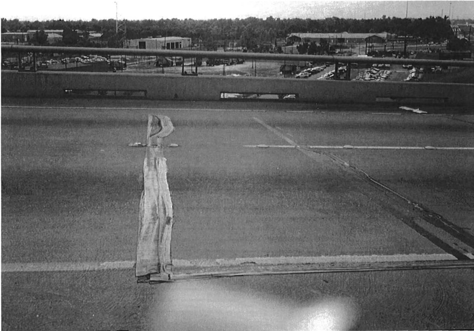
Figure 2-6. Deformed Piezo Sensors at Location C
