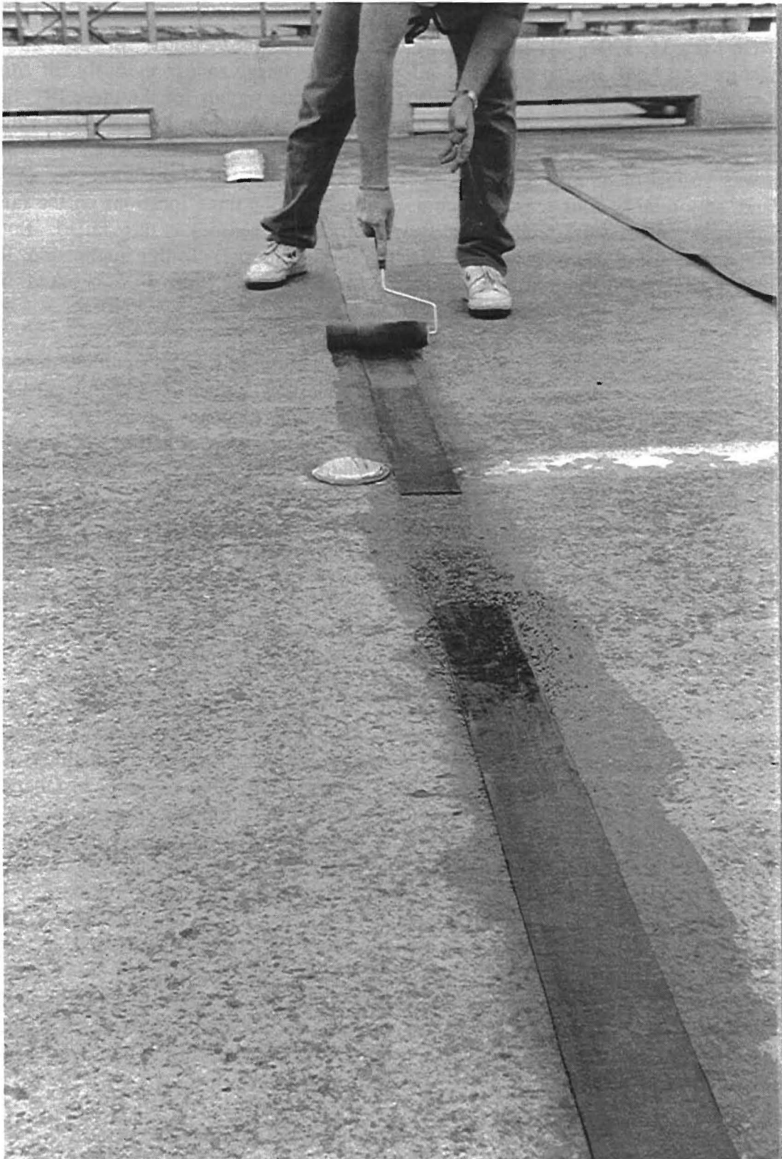
Figure 2-1. Applying Polygard and Primer for Piezo Sensors
