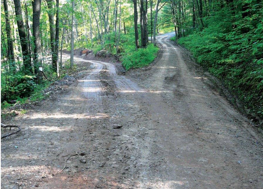
These unpaved gravel roads in the vicinity of oil pad well sites in Lycoming County, PA, show deterioration and rutting along the shoulders.
