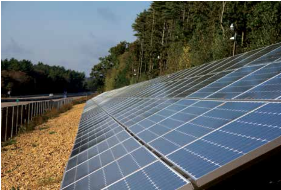
The Massachusetts DOT placed this solar array alongside State Route 44 near Carver, putting the solar panels into service in October 2012. The 99-kilowatt system provides electricity to a nearby water treatment facility. Photo: Gina Filosa, Volpe Center.
