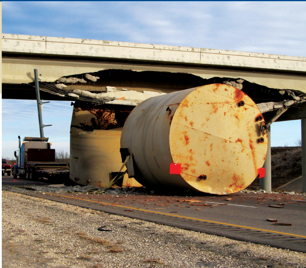
A truck transporting a load of oil field storage tanks struck this overpass bridge on I-10 in Pecos County, TX, about 8 miles (12.8 kilometers) east of Bakersfield. Impacts, such as bridge strikes, to roadway infrastructure from activities related to energy development are the focus of the NCHRP Synthesis 469. Photo: Texas Department of Transportation.
