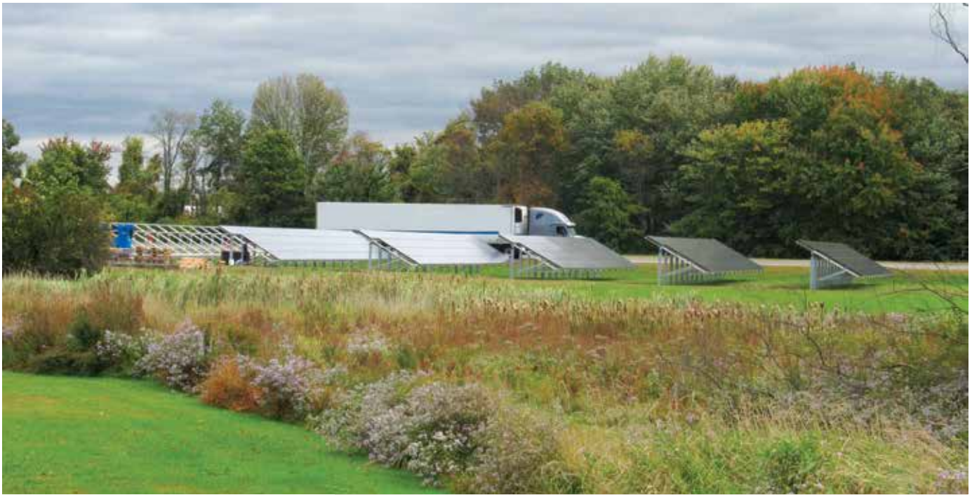
This 325-panel solar array located along I-91 in Northampton, MA, generates approximately 70 kilowatts of power, which offsets energy demand from a nearby office building. Photo: Daryl Amaral, Massachusetts DOT.
