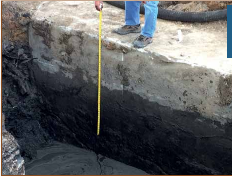
Excavation of the material above and alongside the pier 13 footing shows shear cracks (seen here near the end of the tape measure).
