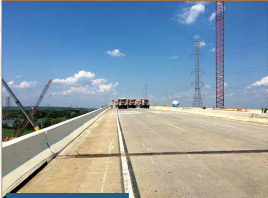
As a load test, these six (two rows of three) loaded dump trucks are stopped on the completed, leveled superstructure, which is supported solely on the temporary towers.
