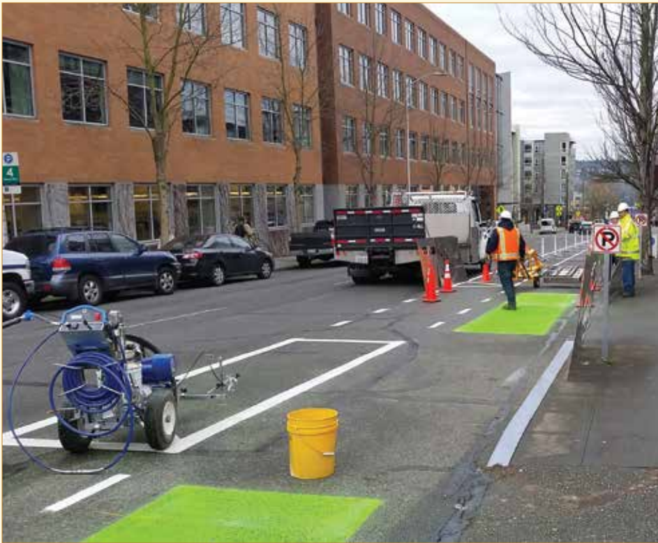
(Left) FHWA supports the installation of well-designed, well-connected bicycle facilities. Protected bike lanes are physically separate from vehicles and are distinct from the sidewalk. Here, the Seattle Department of Transportation is adding a protected bike lane on the west side of Roosevelt Way, NE. Photo: Seattle Department of Transportation.
