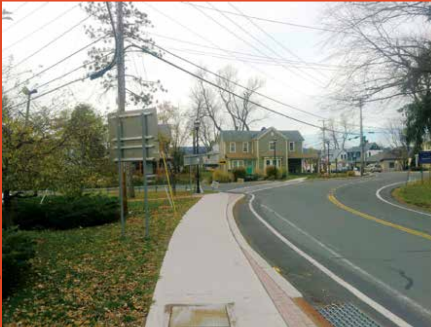
(Before, top) Previously, the entrance to Gardiner, NY, along Route 44/55 Main Street had a broad shoulder but no pedestrian accommodation. (After) The New York State Department of Transportation (NYSDOT) narrowed the shoulder to install a curb and sidewalk to improve pedestrian access.
