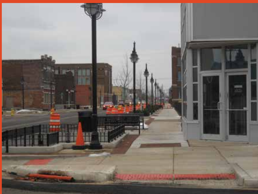
(Before, top) In Peoria, IL, this sidewalk at the intersection of Elm Street and Adams Street was inaccessible. (After) The city reconstructed and widened the sidewalk to provide an ADA-compliant curb ramp for each crosswalk. Street lamps were also installed as part of the project.
