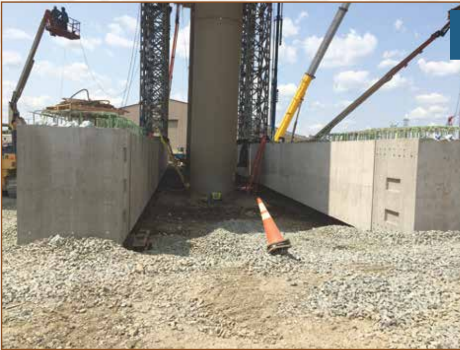
Grade beams shown here were cast on top of drilled shafts.
