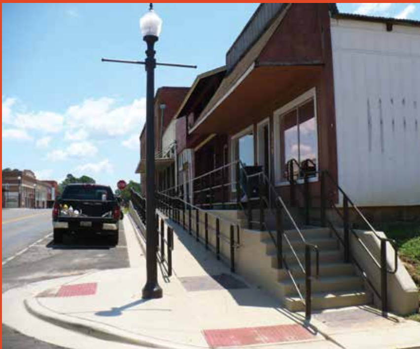
(Before, top) To access the elevated sidewalk and entrances to these businesses near the intersection of SH-11 and Taylor Street in Linden, TX, visitors had to climb this flight of stairs. (After) The Texas Department of Transportation (TxDOT) installed a split sidewalk providing both ramp and stair access to the sidewalk and businesses.
