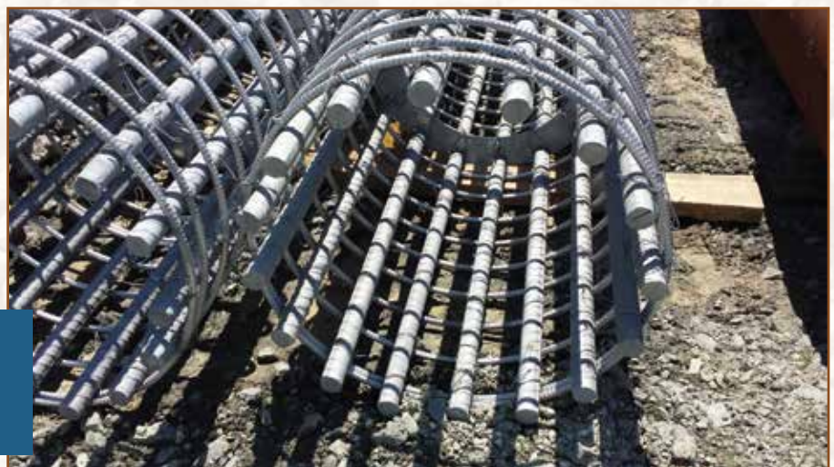
Officials with New York's Tappan Zee Bridge project provided DelDOT with these reinforcing steel cages for the drilled shafts.
