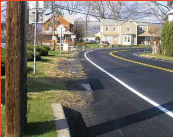
(Before, top) Previously, the entrance to Gardiner, NY, along Route 44/55 Main Street had a broad shoulder but no pedestrian accommodation. (After) The New York State Department of Transportation (NYSDOT) narrowed the shoulder to install a curb and sidewalk to improve pedestrian access.
