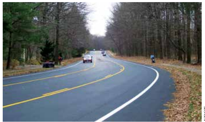
A road diet implemented along this stretch of Soapstone Drive in Reston, VA, changed the configuration from two lanes in each direction to the three lanes shown here and reduced crashes by 65 percent.
