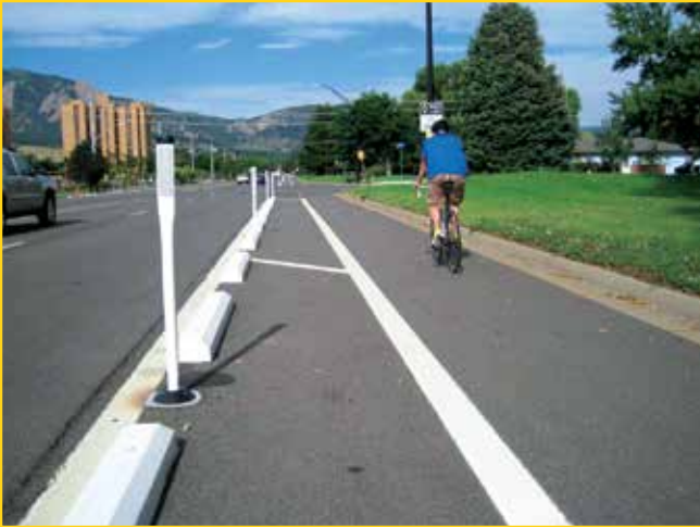
(Above) This one-way bicycle lane in Boulder, CO, is separated from the roadway by a series of parking stops and delineator posts.
