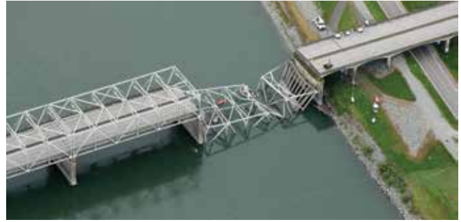
WSDOT's Bridge Vertical Clearance Trip Planner helps truck drivers research bridge heights to avoid potential conflicts, such as the overheight impact from a commercial truck that caused this section of the Skagit River Bridge in Mount Vernon, WA, to collapse in May 2013.
