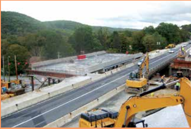
The New York State DOT used accelerated bridge construction techniques to erect two bridges on I-84 over Dingle Ridge Road in southeast Putnam County in just two weekends. The project leveraged research from SHRP2 and FHWA funding to minimize delays to motorists on this major route between New York and Connecticut.
