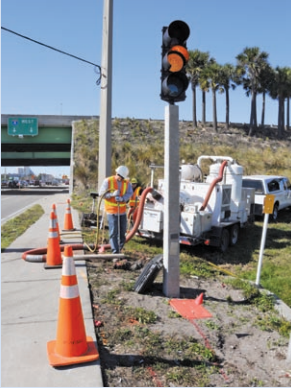
A worker loosens soil with an air lance in preparation for excavating a test hole.
