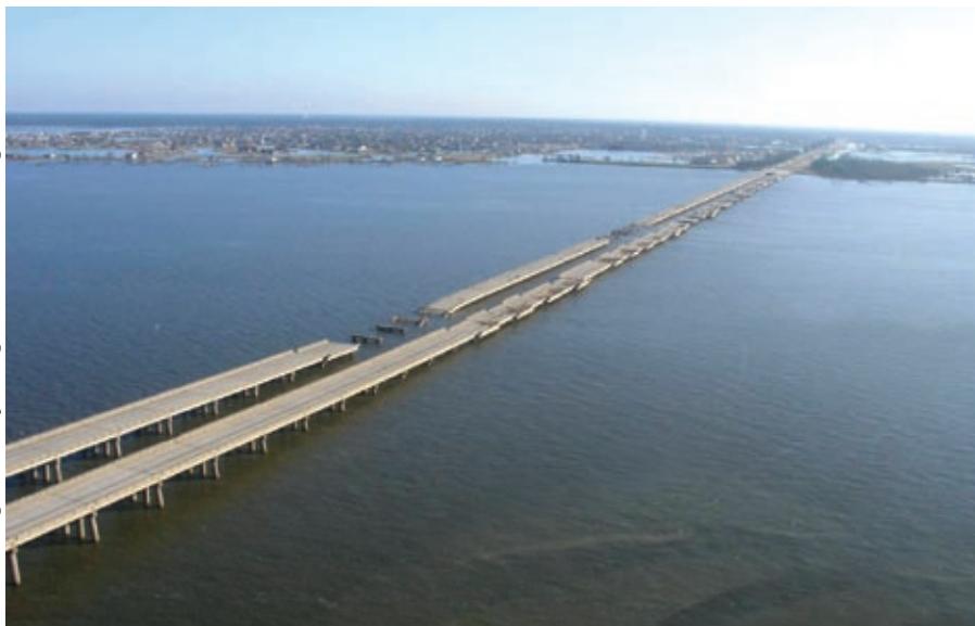
Wave-induced forces during Hurricane Katrina lifted and misaligned these multiple spans of the I-10 twin bridges over Lake Pontchartrain.
