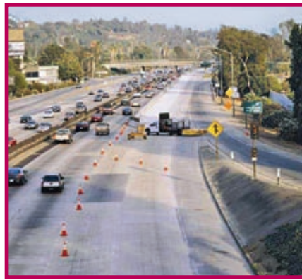
Caltrans has surface-ground this portion of I-10 near Pomona three times, helping extend the life of the heavily traveled route to more than 60 years, without significant reconstruction.
