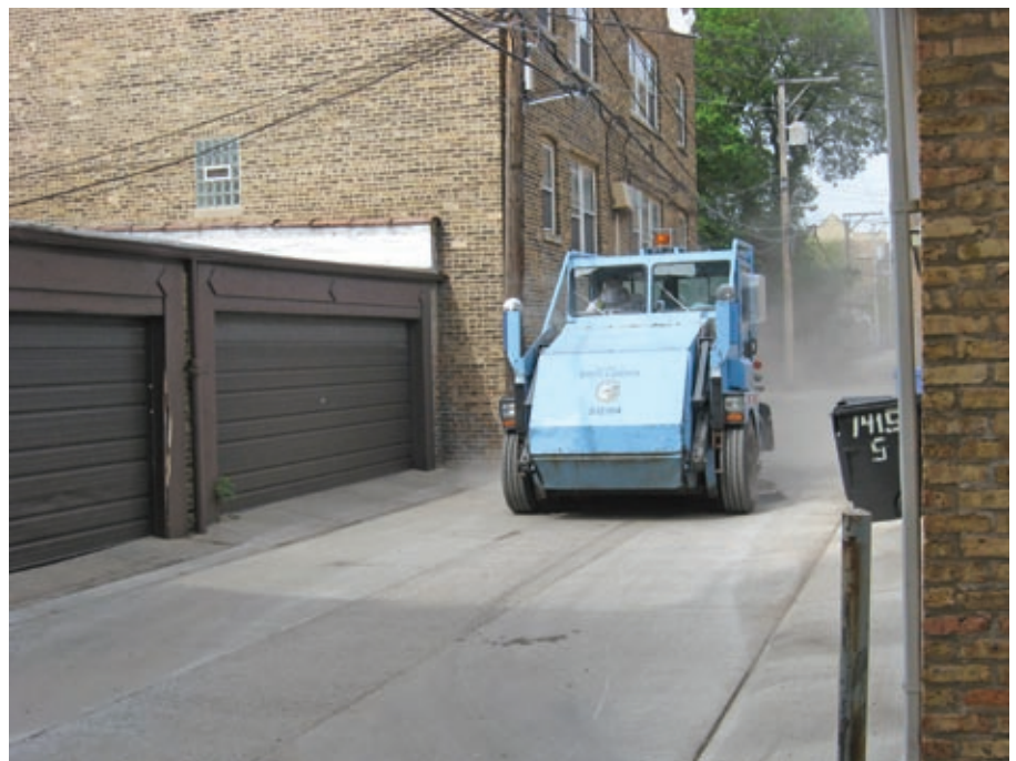
A maintenance worker is using a broom-only streetsweeper to clean the center trench in this alley paved with pervious concrete.
