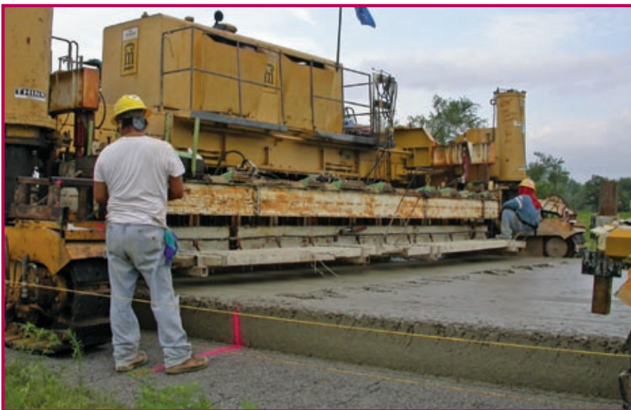
This crew working on I-40 near Checotah, OK, is using a concrete overlay machine outfitted with an automatic dowel bar inserter, which expedites the paving process.
