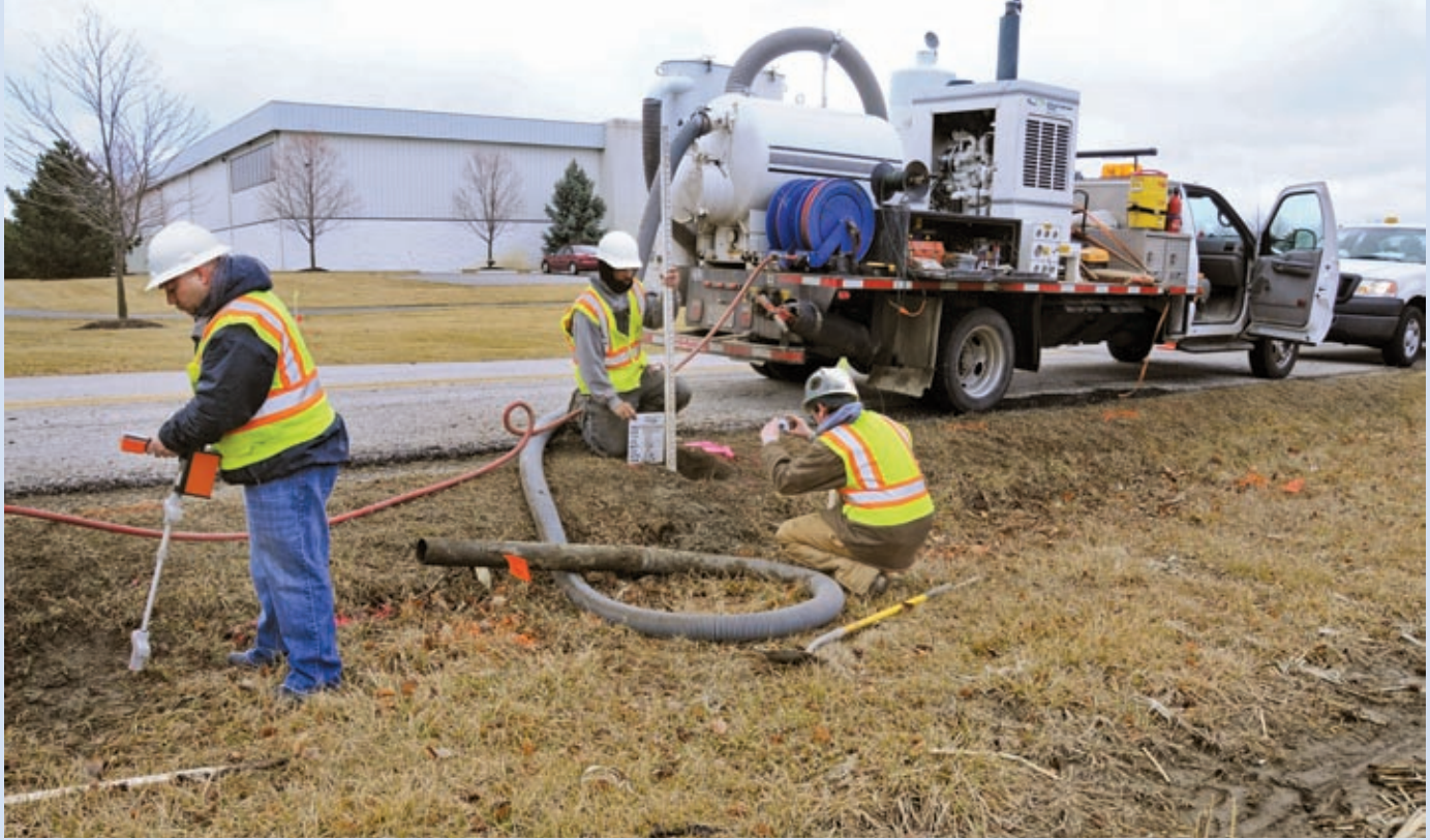
Three SUE technicians are using a pipe and cable locator and nondestructive vacuum excavation to locate subsurface utilities. After exposing the utilities, the workers survey and record information pertinent to the type of utility and its size, depth, and condition. The workers record the data both electronically and on a poster board, which they photograph (as shown here) for quality assurance purposes.
