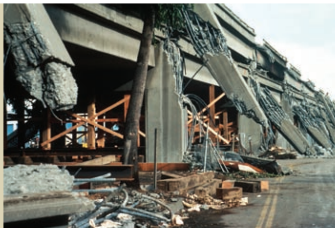
Side view of support-column failure and a collapsed upper deck of the Cypress Freeway in the San Francisco Bay area after the 1989 Loma Prieta earthquake.
