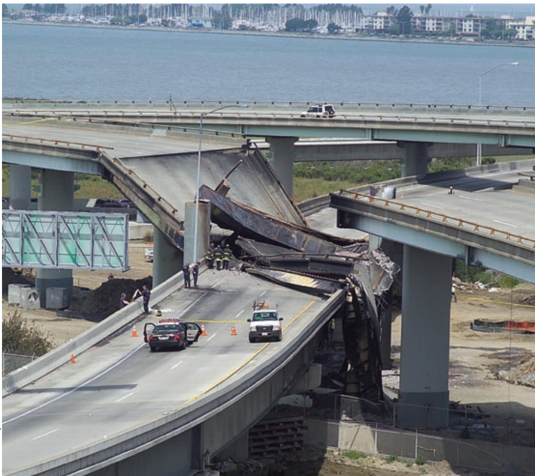
In the San Francisco Bay area, CA, on April 29, 2007, a tanker truck crash and explosion created a gaping hole in the "MacArthur Maze." This portion of the I-80 eastbound to I-580 eastbound connector ramp collapsed onto I-80 westbound and the I-880 southbound connector ramp.
