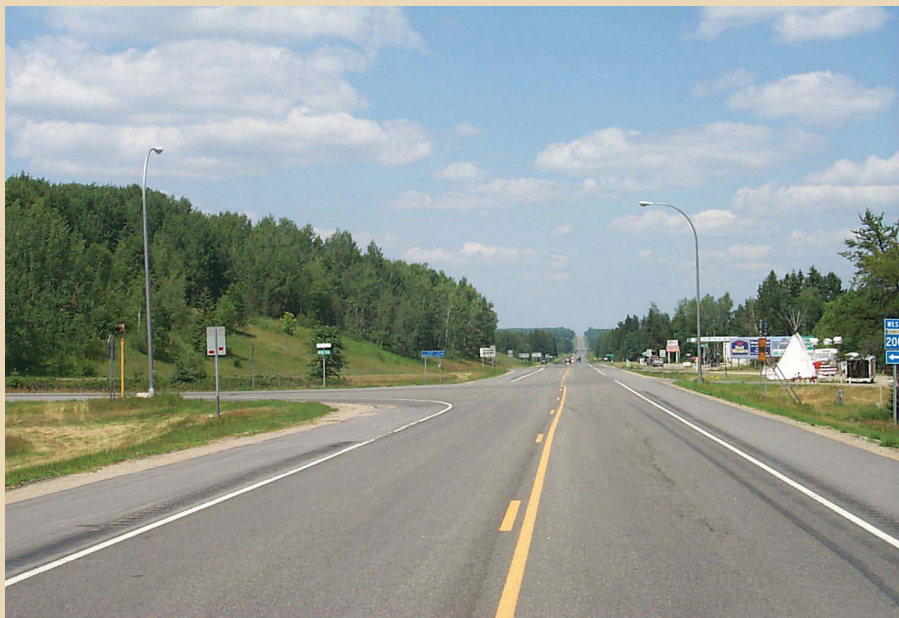
Installation of street lighting at this rural Minnesota intersection helped to stop a pattern of nighttime fatal and injury crashes.
