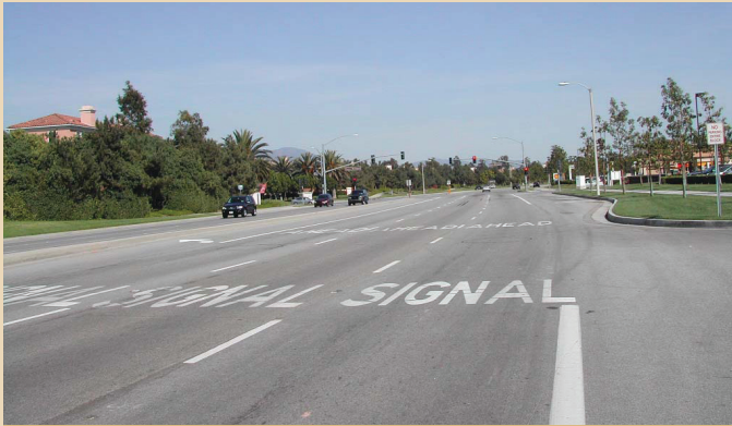
Traffic messages painted on the pavement in the driving lane, in full view of oncoming motorists, can provide an extra measure of communication with the driver. (Left) Motorists are alerted to an upcoming signal in Irvine, CA. (Right) Route markers on the pavement approaches to this intersection in Orlando, FL, help guide motorists to interstate access.
