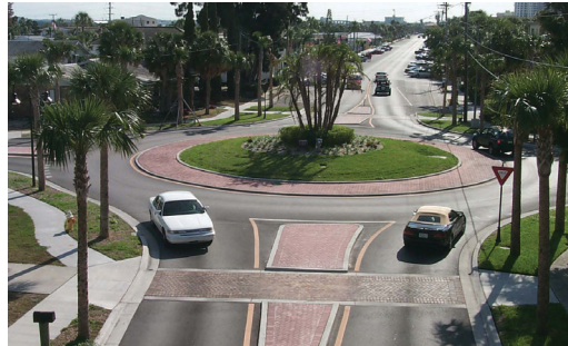
Typical circulating speeds in Clearwater's four one-lane roundabouts such as this one are 18 to 21 kph (11 to 13 mph), and typical approach speeds (measured at the crosswalks) are 23 to 26 kph (14 to 16 mph). Photo: Ken Sides, City of Clearwater, FL.
