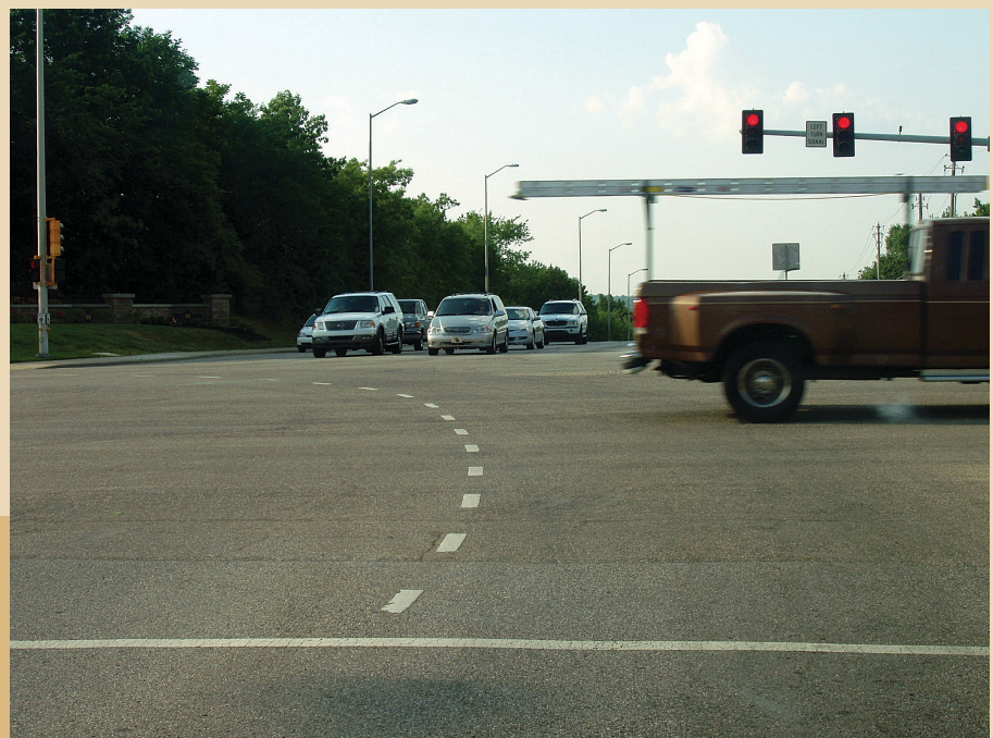
The extension of left-turn lane markings into an intersection, shown here in Overland Park, KS, is a common treatment to help guide multiple lanes of turning traffic through intersections.
