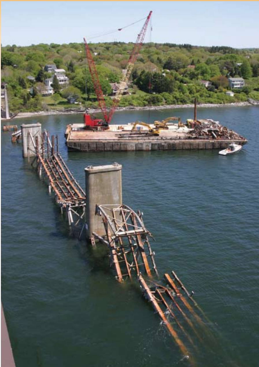
A construction barge is approaching the old bridge to salvage the steel for recycling.
