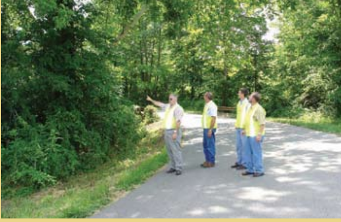
Between 2000 and 2005, 13 crashes were reported along this stretch of New Cummer Road in Morgan County. In 2005, county transportation officials dramatically improved safety along a bridge approach by clearing trees and brush to improve sight distances in the approach curve and installing Type 3 object markers to mark the bridge corners.
