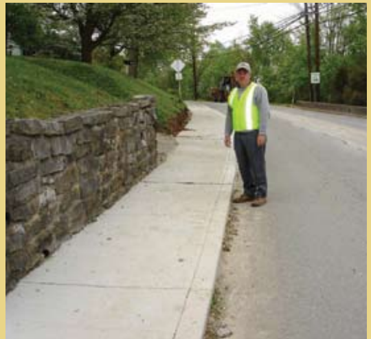
Pulaski County, KY, replaced 762 linear meters (2,500 feet) of sidewalk along Jacksboro Road in the city of Somerset. Top: The old sidewalk was at the same level, or even lower, than the roadway. Bottom: The new sidewalk, which is elevated above the level of the roadway, improves pedestrian safety along this road.
