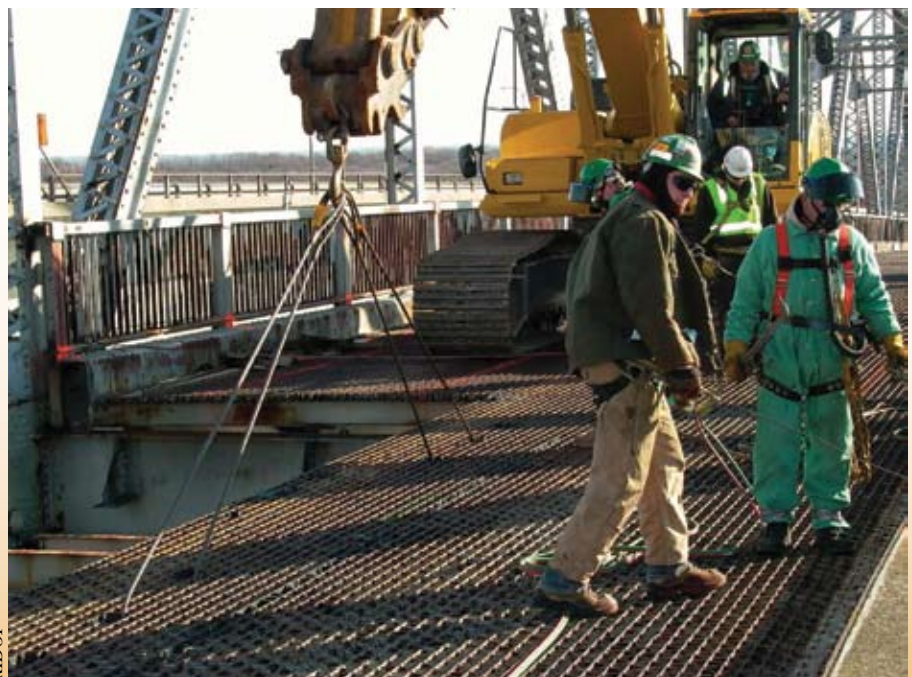
These workers are removing the deck of Old Jamestown Bridge during the preparatory work that preceded the first demolition.
