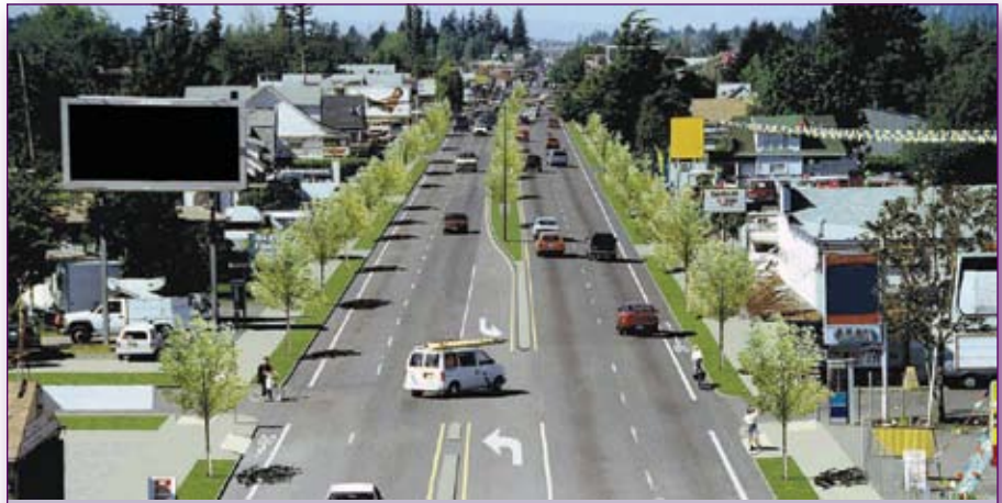
A digital illustration superimposed upon this photograph provides an example of how simple changes—access management, a raised median, bicycle lanes, sidewalks, and landscaping—can make the roadway environment more safe and appealing for pedestrians. Photo: Michael Ronkin, Designing Streets for Pedestrians and Bicyclists .
