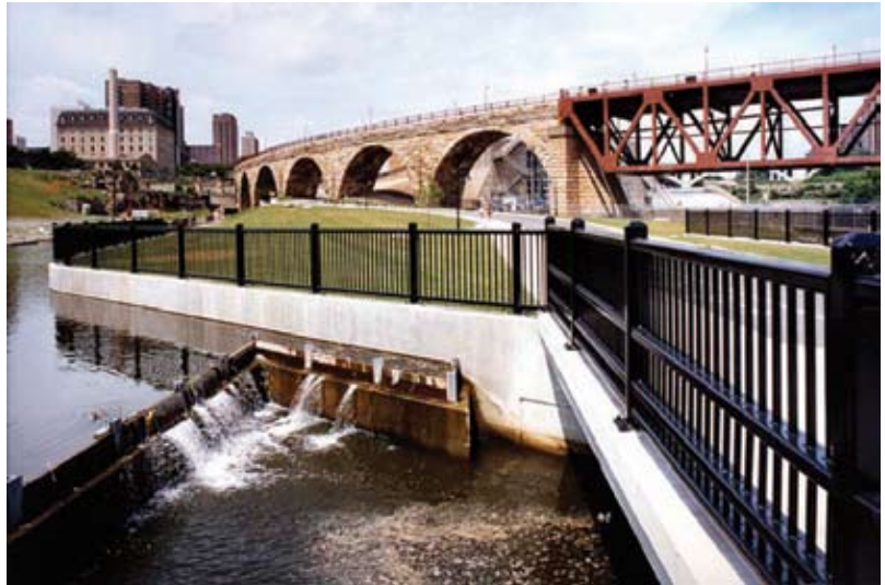
NHI's courses on historic preservation and water quality management of highway runoff will help transportation professionals comply with associated regulations and create balance between project delivery and stewardship of historic properties such as the Mills Ruins Park, shown here, in Minneapolis, MN.
