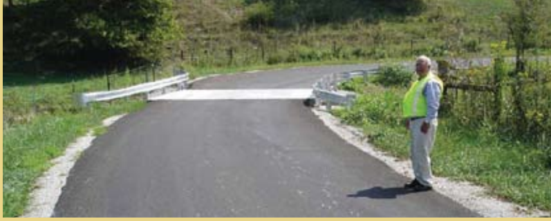
Mason County widened this small bridge along Cliff Pike Road and added guardrails to improve safety.
