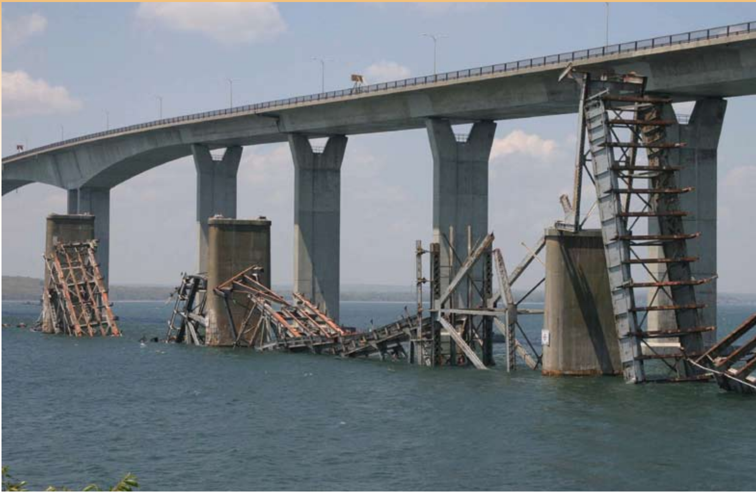
The new bridge dwarfs the remains of the old one. Photo: RIDOT.
