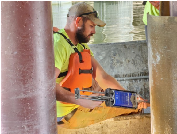
Figure A.19: Applying Epoxy to Joint
