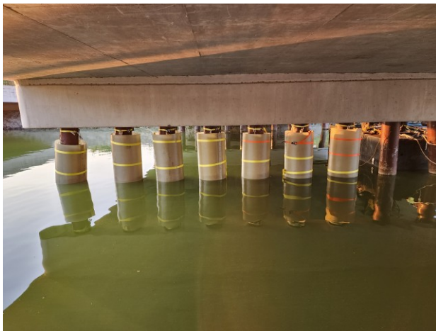
Figure A.14: North Pier Pile Jackets Ready for Grout
