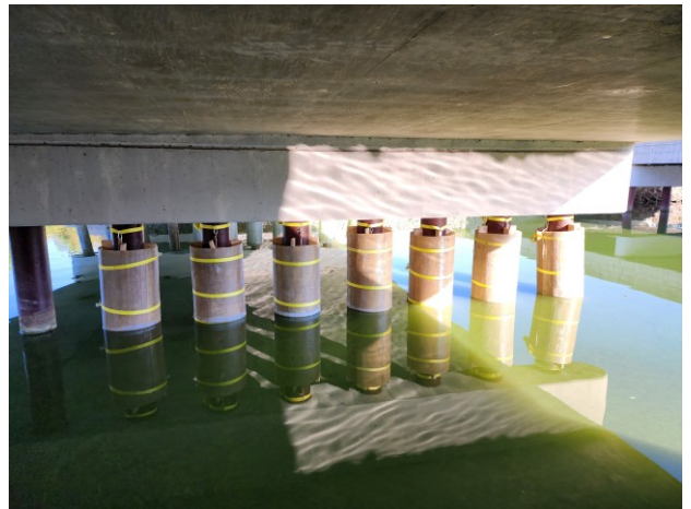
Figure A.22: South Pier Pile Jackets Ready for Grout
