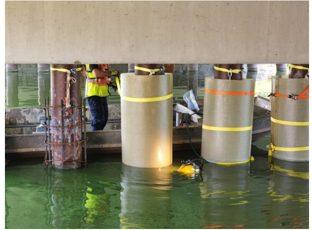
Figure A.10: Placing Straps Around Jacket
