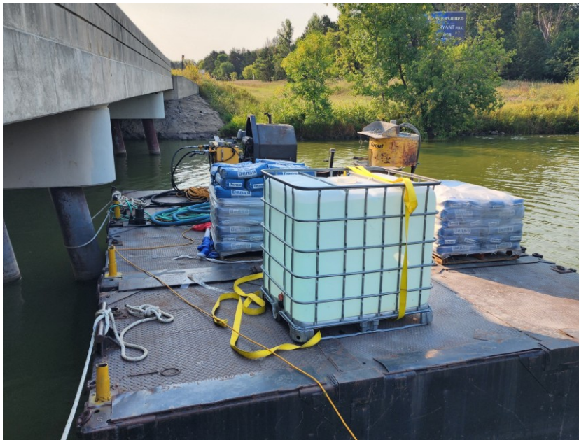
Figure 3.11: Grouting operation on the barge
