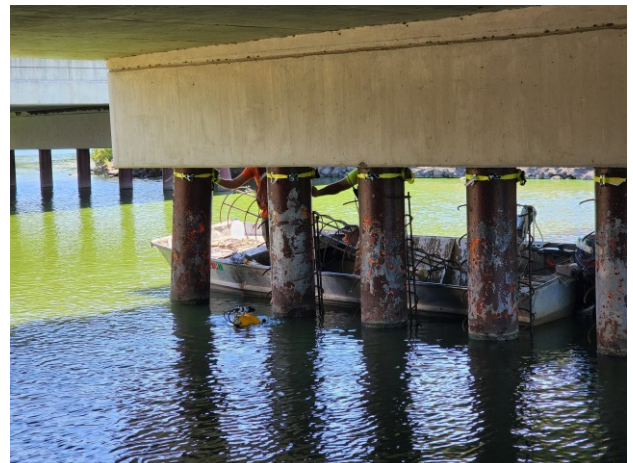
Figure A.5: Placing Rebar Cage
