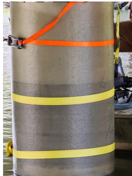
Figure A.17: Water Level Rising in Jacket During Grouting Operation
