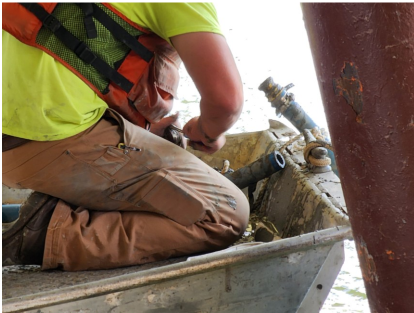
Figure 3.19: Grout line connection came apart
