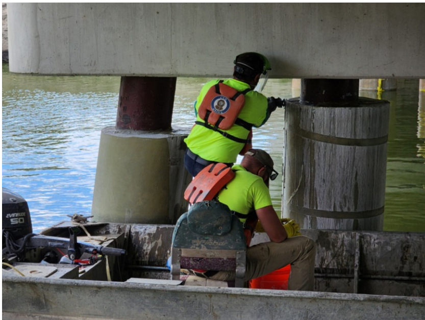
Figure 3.13: Trimming top of jacket
