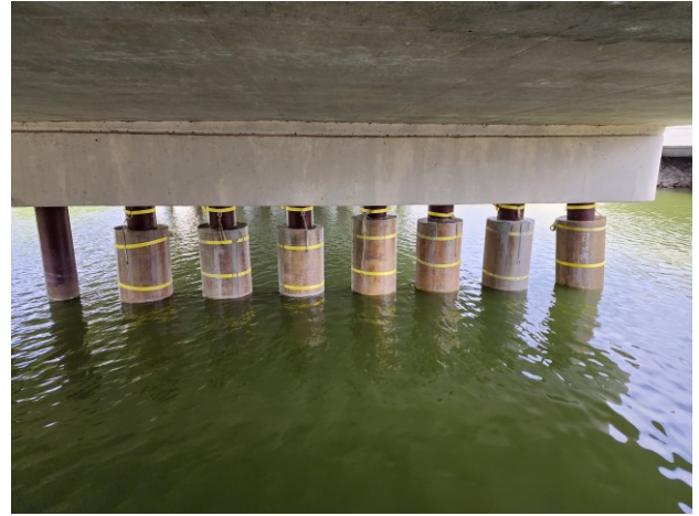
Figure A.32: South Pier without Splash Zone
