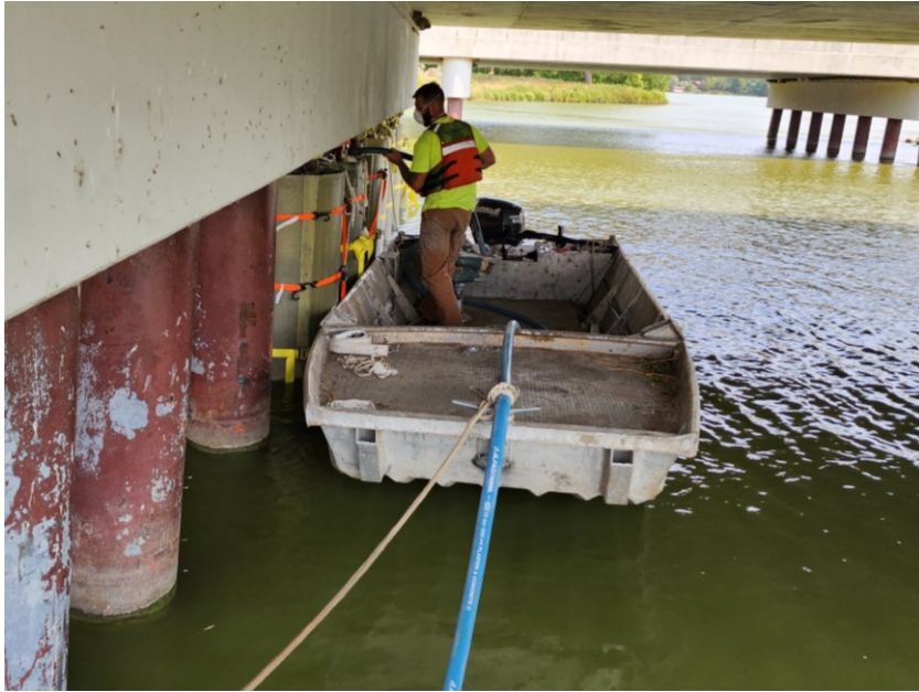
Figure 3.12: Pumping grout into jacket
