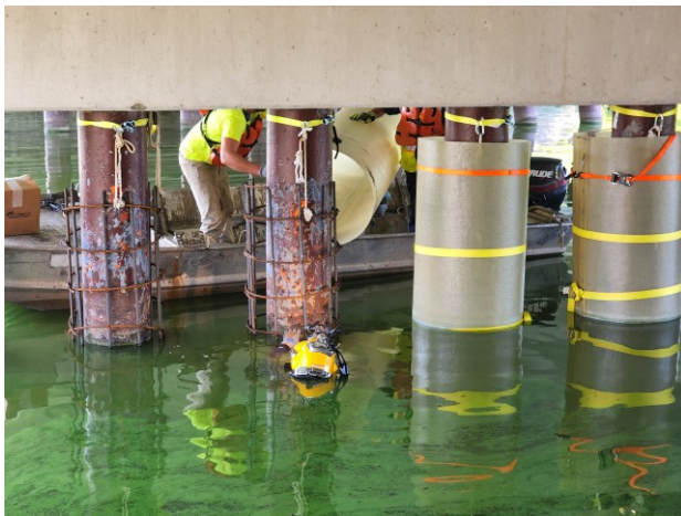
Figure A.8: Placing Pile Jacket
