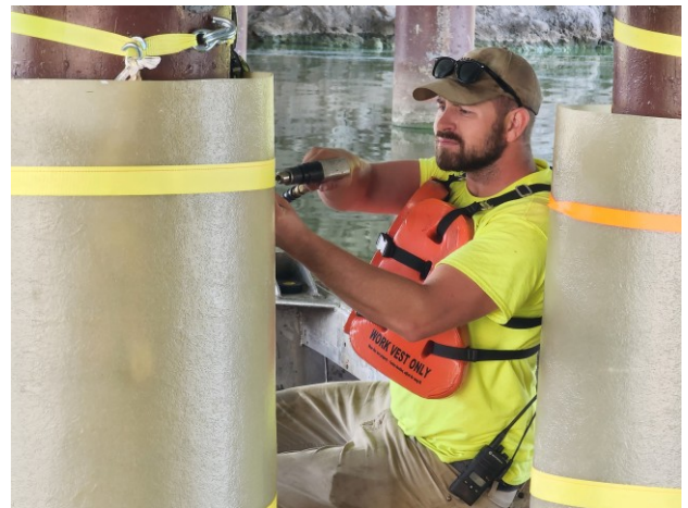
Figure A.11: Installing Screws
