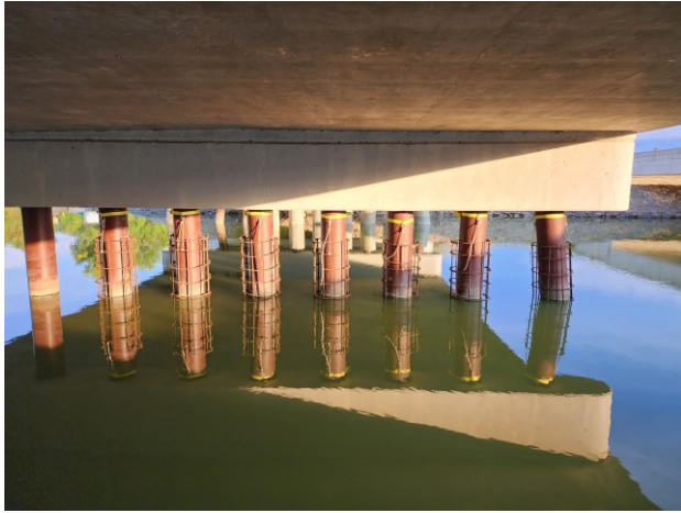
Figure A.18: South Pier with Reinforcement Hanging
