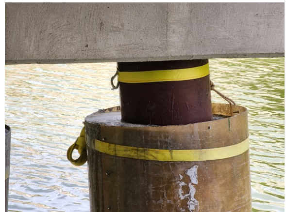
Figure A.33: South Pier Eastern Most Pile Without Splash Zone
