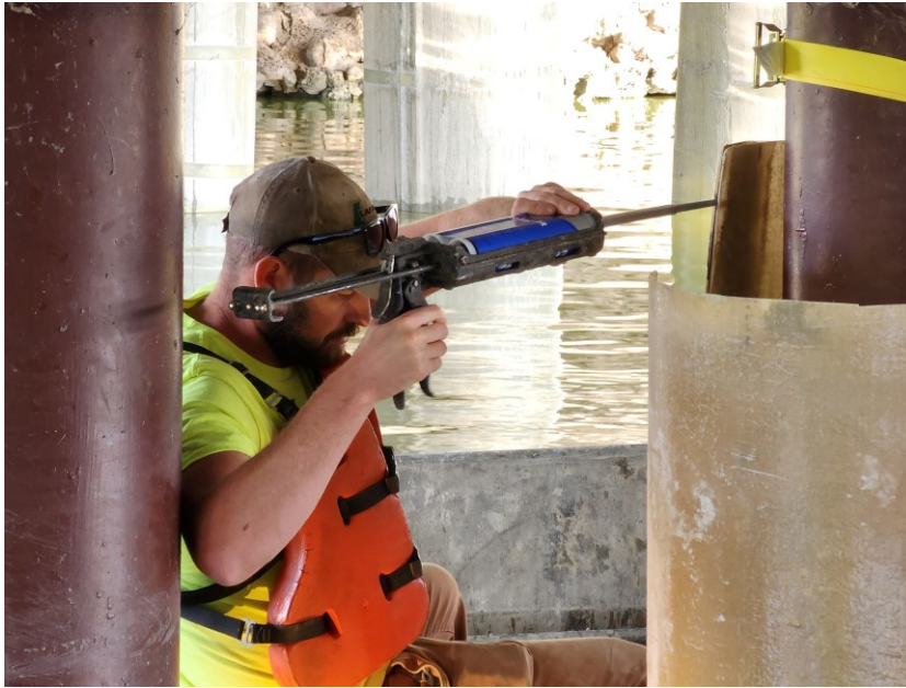
Figure 3.6: Worker in boat applying epoxy to tongue-and-groove joint above water
