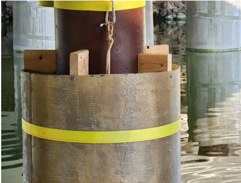
Figure 3.9: Wood spacers at top of jacket
