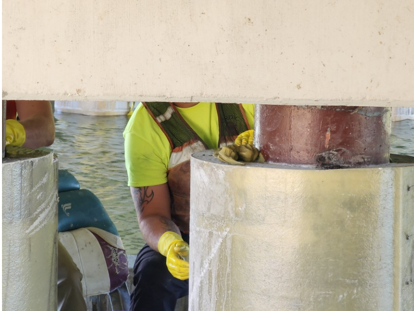
Figure 3.14: Epoxy ball on top of grout before being spread out
