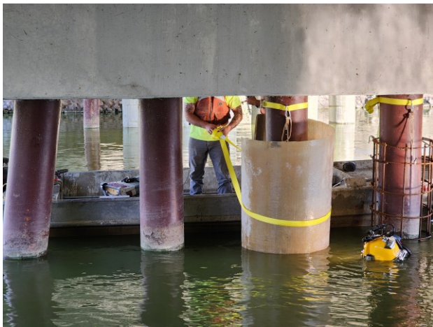
Figure A.20: Placing Straps on Five Star Jacket
