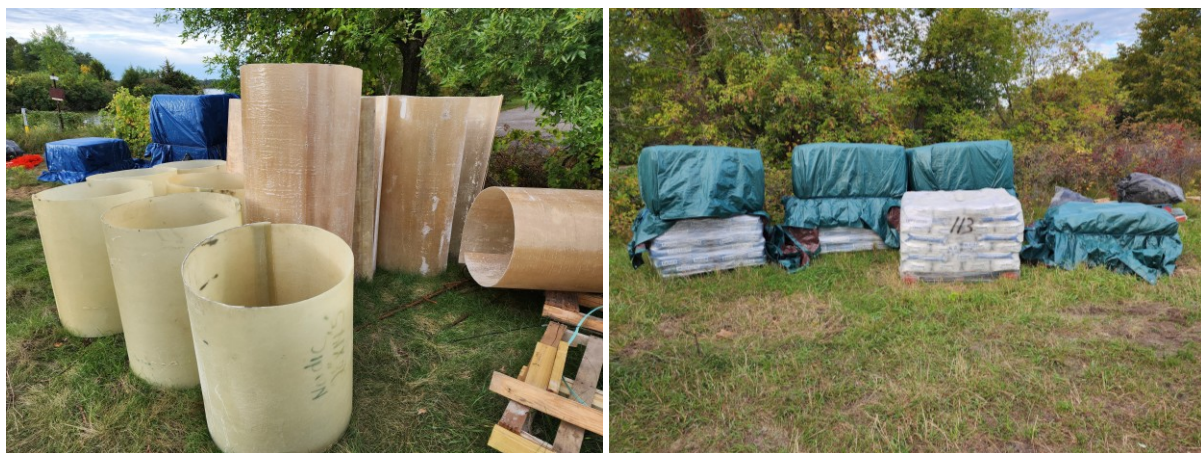
Figure 4.1: Scrap Pile Jackets (Left) & Left Over Five Star Grout (Right)
