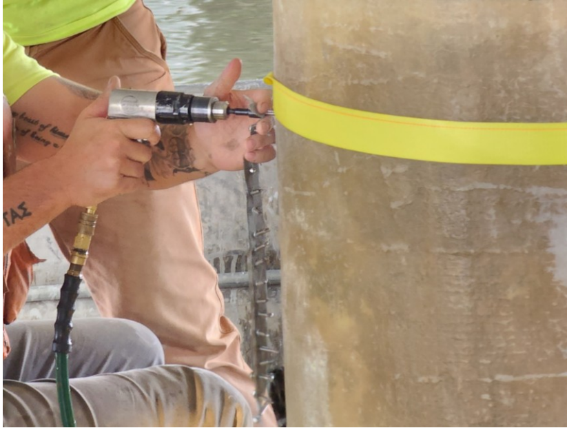
Figure 3.18: Duct tape with screws
