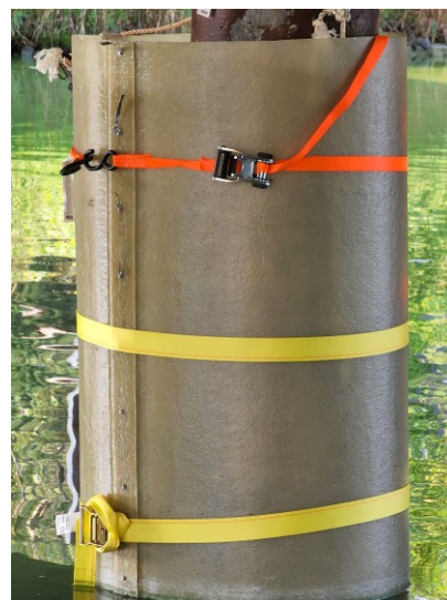
Figure A.12: Installed Jacket Close-up
