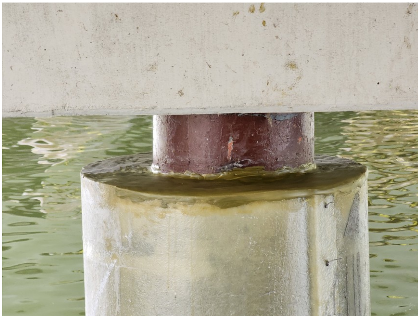
Figure 3.15: Finished jacket with Splash Zone epoxy at the top
