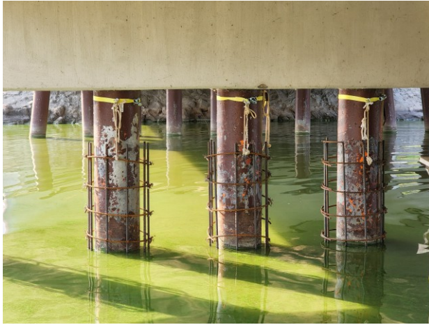
Figure A.7: Reinforcement Hanging from Piles
