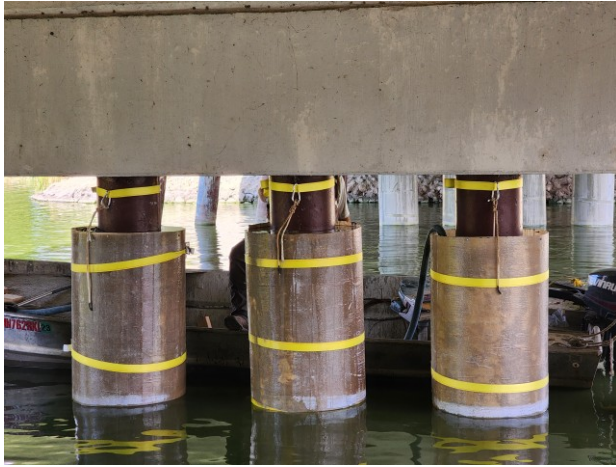
Figure A.23: Grouting on South Pier
