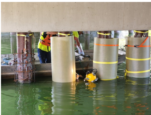
Figure A.9: Apply Epoxy to Joint
