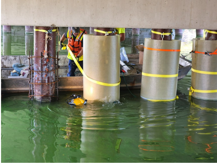
Figure 3.7: Placing ratchet straps around jacket
