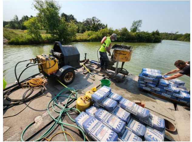
Figure A.16: Grouting Operation on Barge
