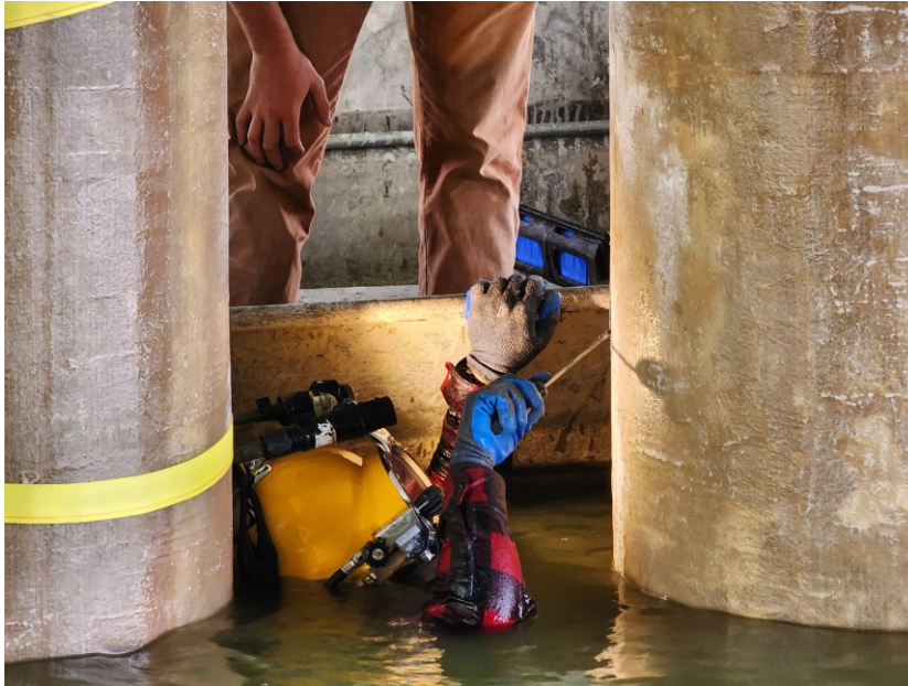
Figure 3.17: Diver using screwdriver on Five Star joint
