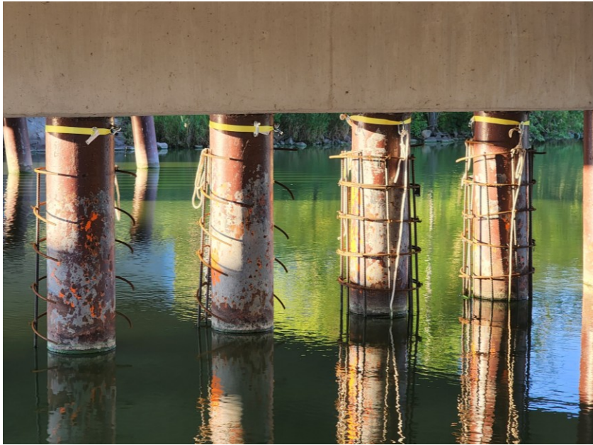
Figure 3.4: Pier 2 (North) reinforcement cages
