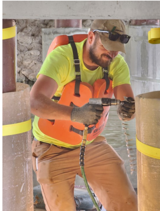
Figure A.21: Installing Screws in Joint
