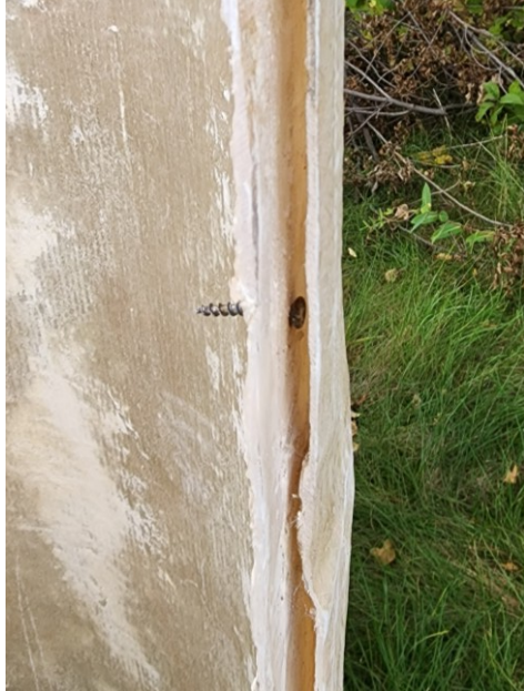
Figure 4.4 Five Star Jacket with screw in joint
