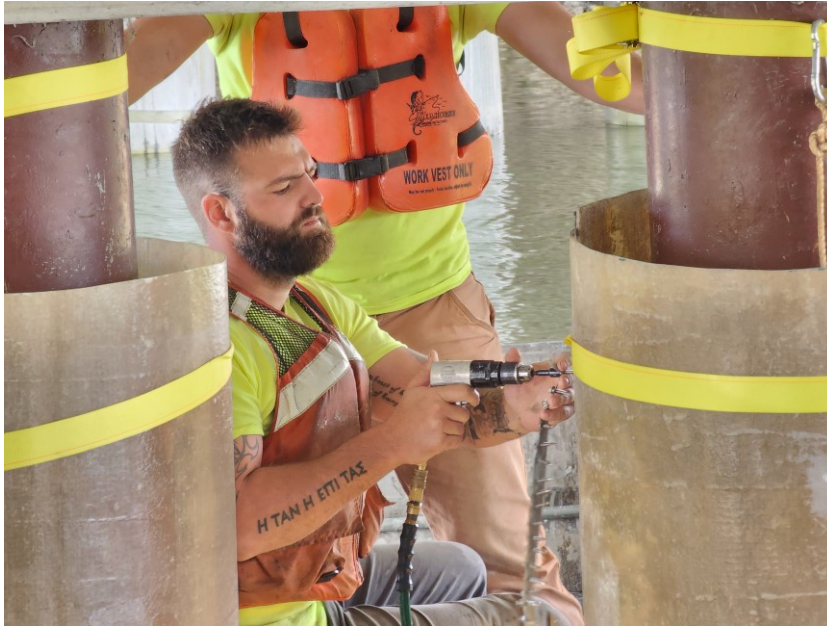
Figure 3.8: Worker securing tongue-and-groove joint with screws
