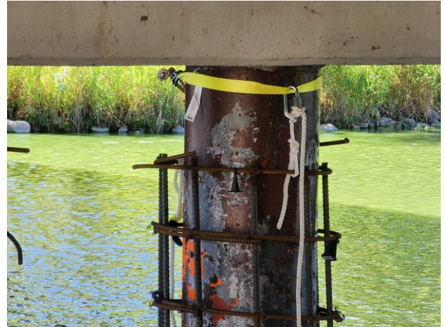
Figure A.4: Close-up of Hanging Rebar
