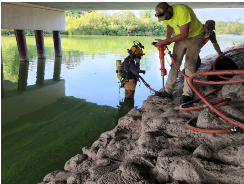
Figure 3.3: Diver prepping to start dive with jackhammer
