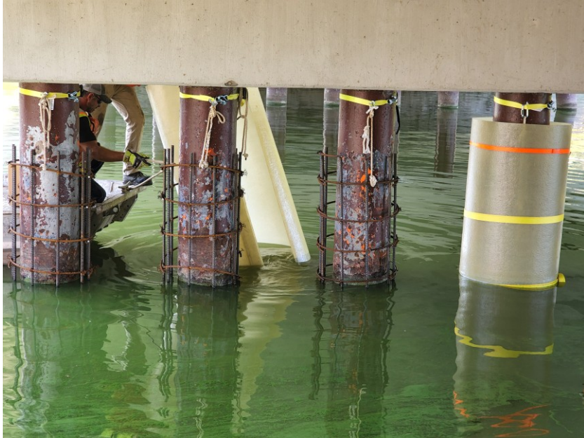
Figure 3.5: Pier 2 (North) Diver opening jacket at the bottom
