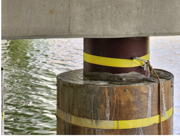
Figure A.35: South Pier 3rd Pile From the East Without Splash Zone
