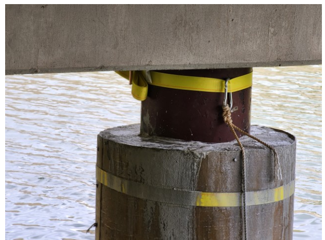
Figure A.34: South Pier 2nd Pile From the East Without Splash Zone
