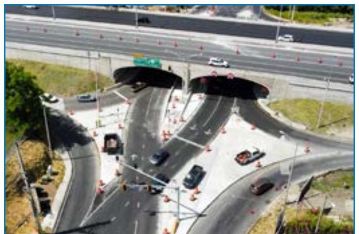
An aerial view of Puerto Rico's first diverging diamond interchange.
