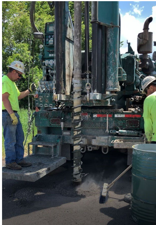
Figure 3.16: Start of HSA drilling at Moore Park
