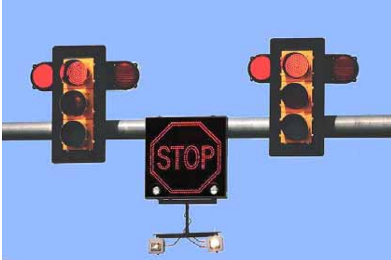
Figure 7. Photo. Warning configuration on the test track.
