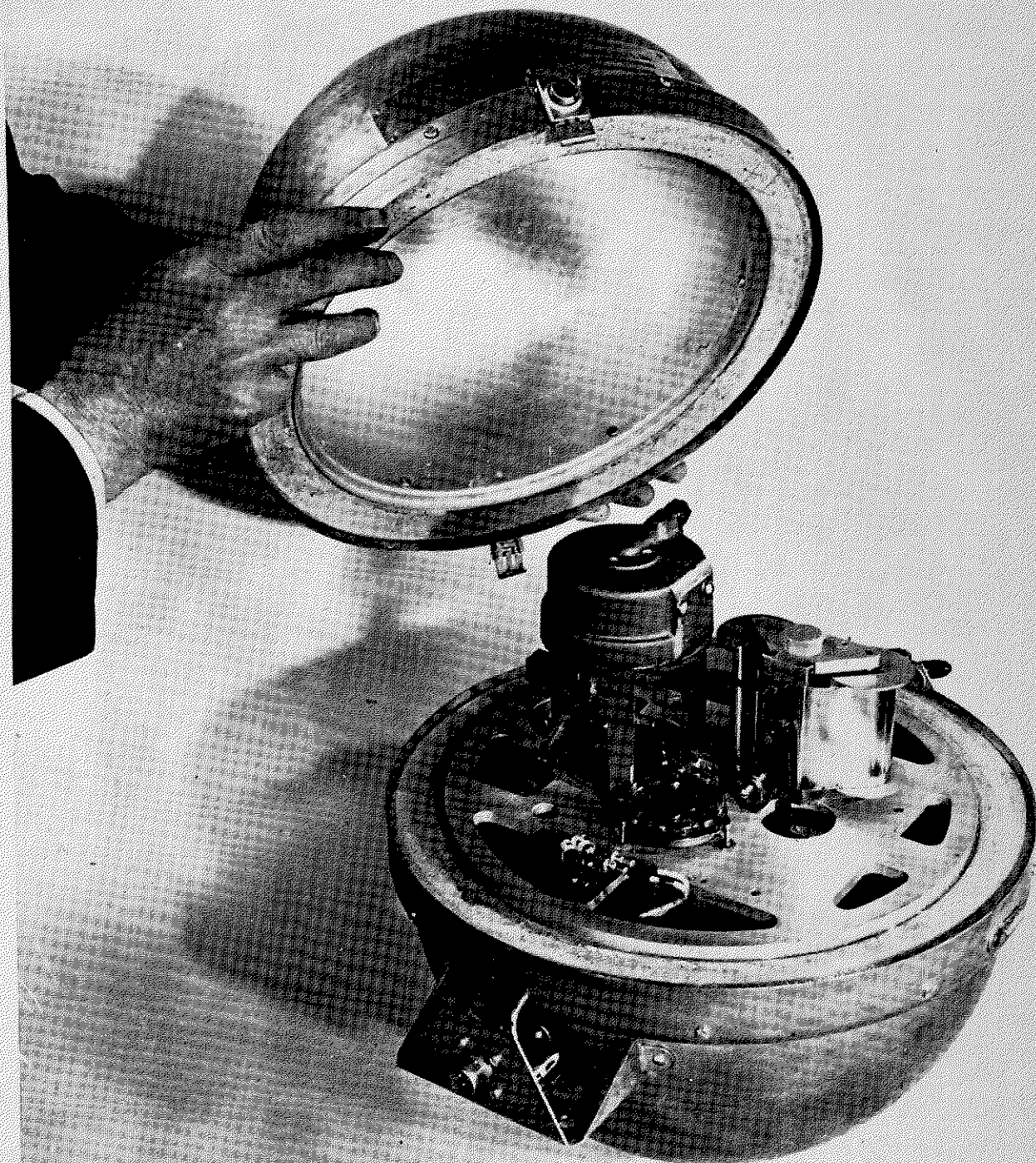
FIG. 1 FLIGHT RECORDER WITH TOP COVER REMOVED
