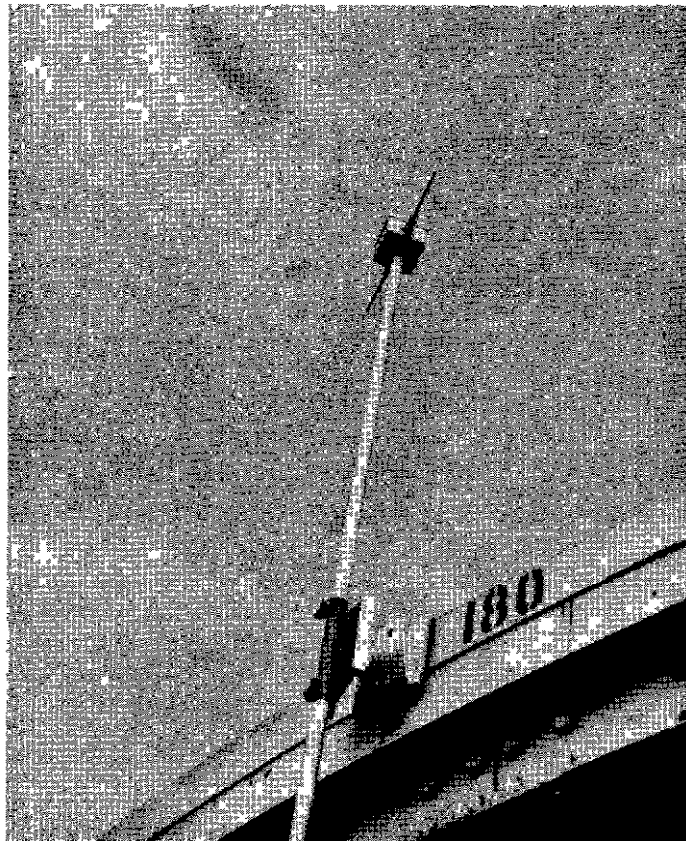
Fig. 1 View of TDEC Counterpoise Detector and Mounting
