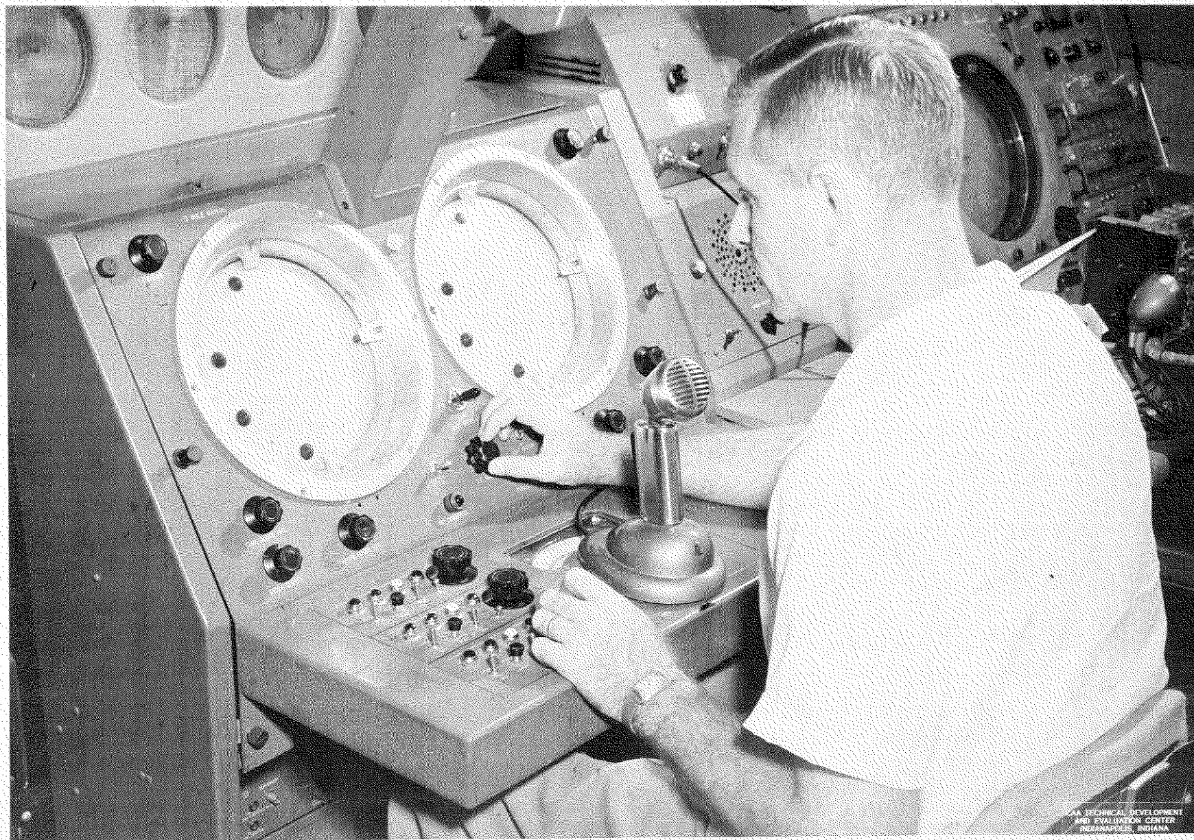
FIG. 2 ARRANGEMENT OF REMOTE CONTROLS FOR PAR-I TRAFFIC CONTROL MONITOR
