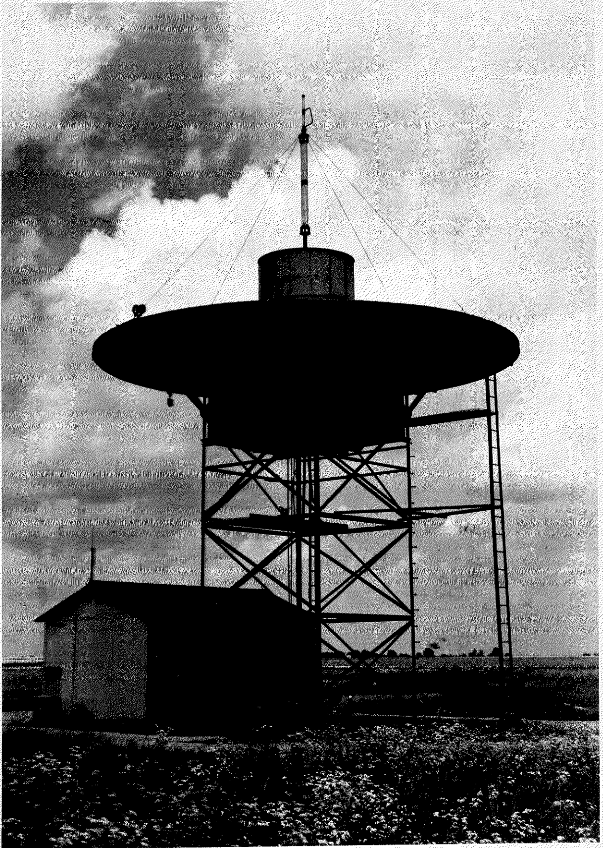
FIG. 10 COMBINED ANTENNA MOUNTED ON OMNIRANGE
