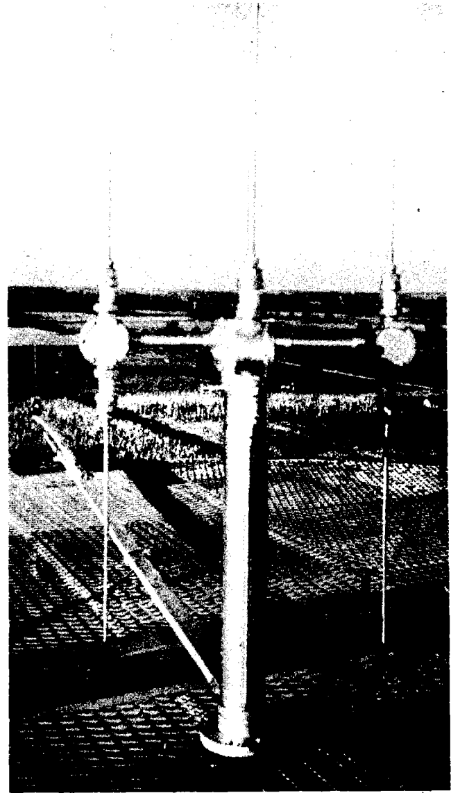
Figure 14. 63-MC Radio Range 4-Course Vertically Polarized Antenna, Indianapolis, Indiana.
