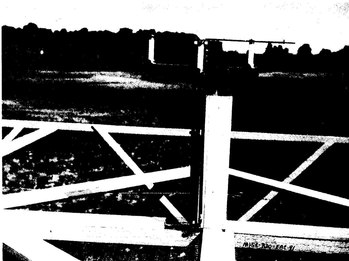
Figure 33. 125-Megacycle Crossed-Dipole Antenna on Top of the Counterpoise at Indianapolis.
