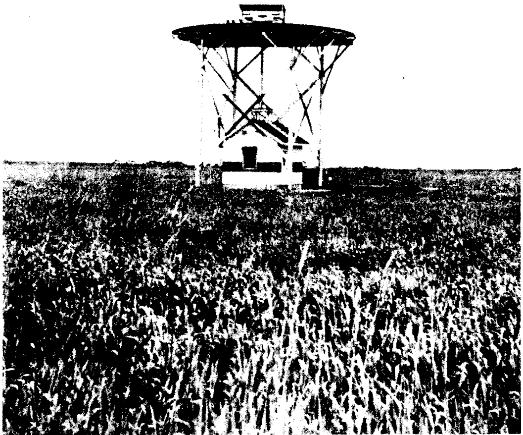
Figure 68. View of the 125-Megacycle Range Station at Indianapolis, Using Pure Horizontally Polarized Ultra-High-Frequency Loop Antennas.
