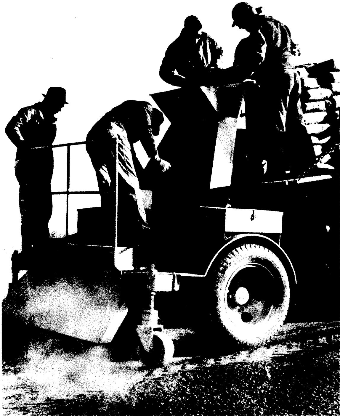
Figure 22. Operation of the Spreader When Using Sacked Cement.
