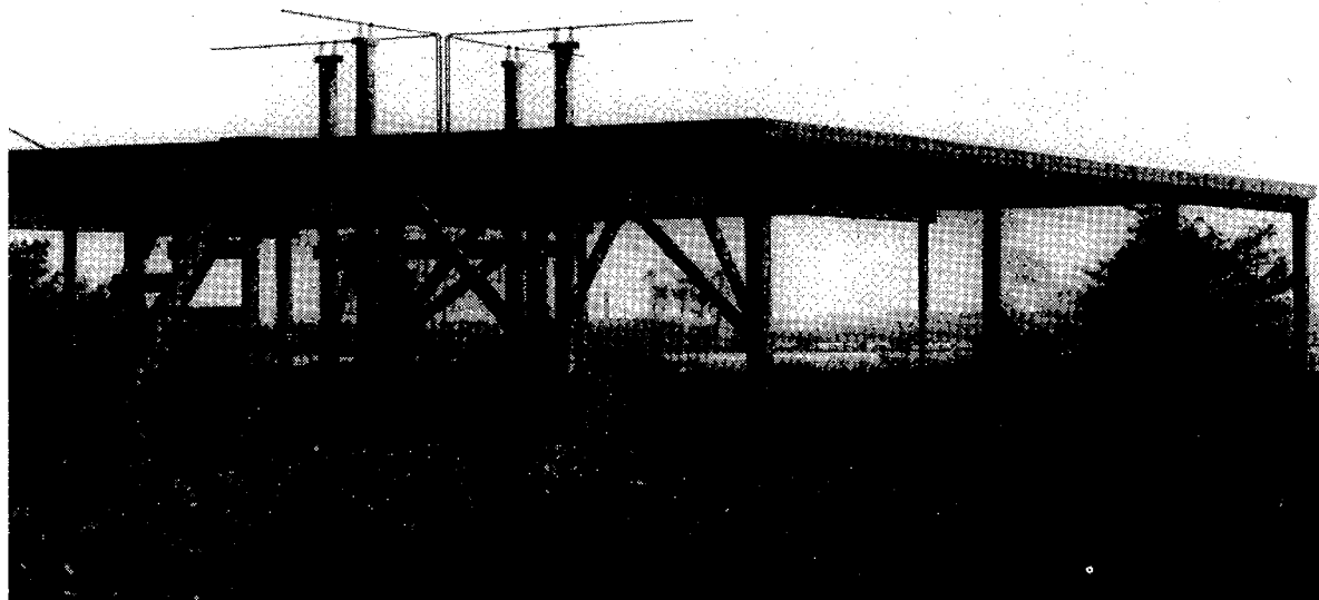
Figure 26.—The experimental counterpoise system as installed at Washington radio range station.
