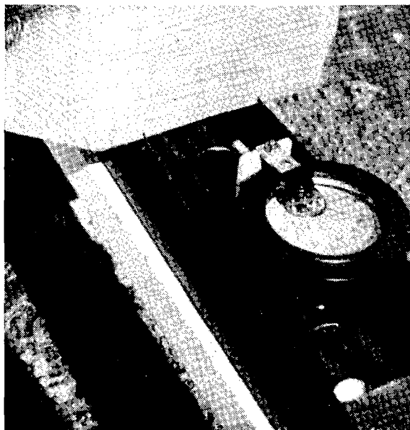
Figure 43.—Spacing block used to secure constant spacing of duct side wall.
