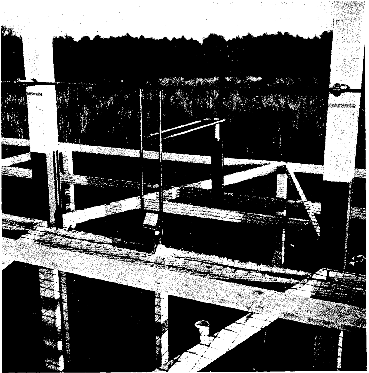
Figure 3.—Showing method adopted for exciting the antenna system, Bowie, Md.
