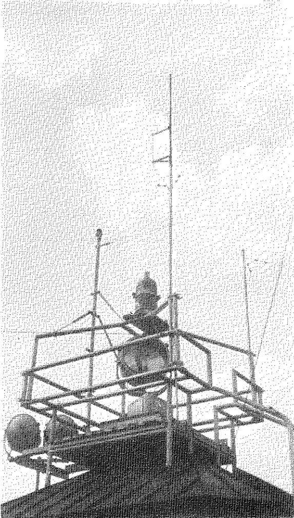
Figure 3.—Vertical antenna installed above control tower.
