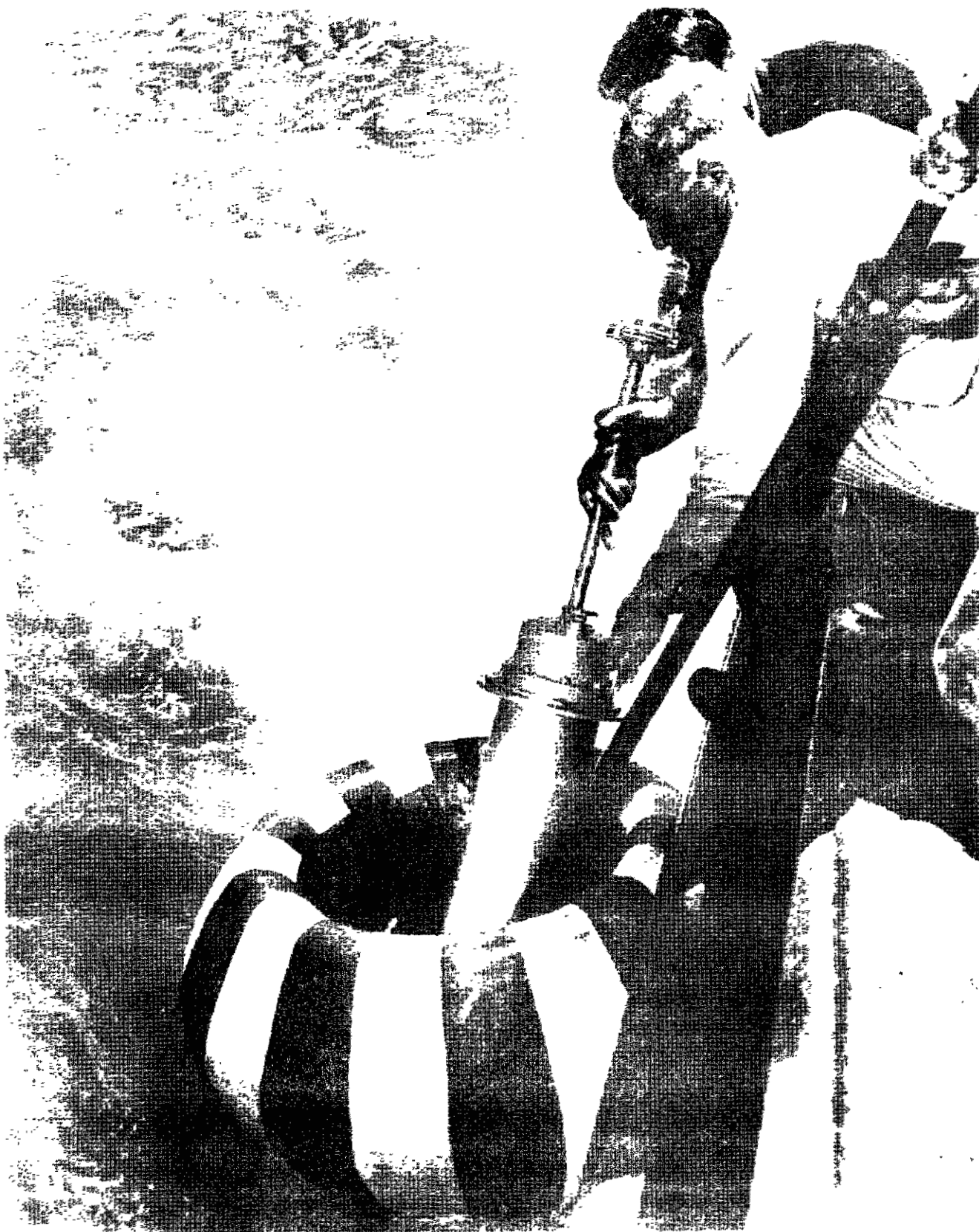
INSTALLING LIGHT UNIT IN RUBBER BUOYS
