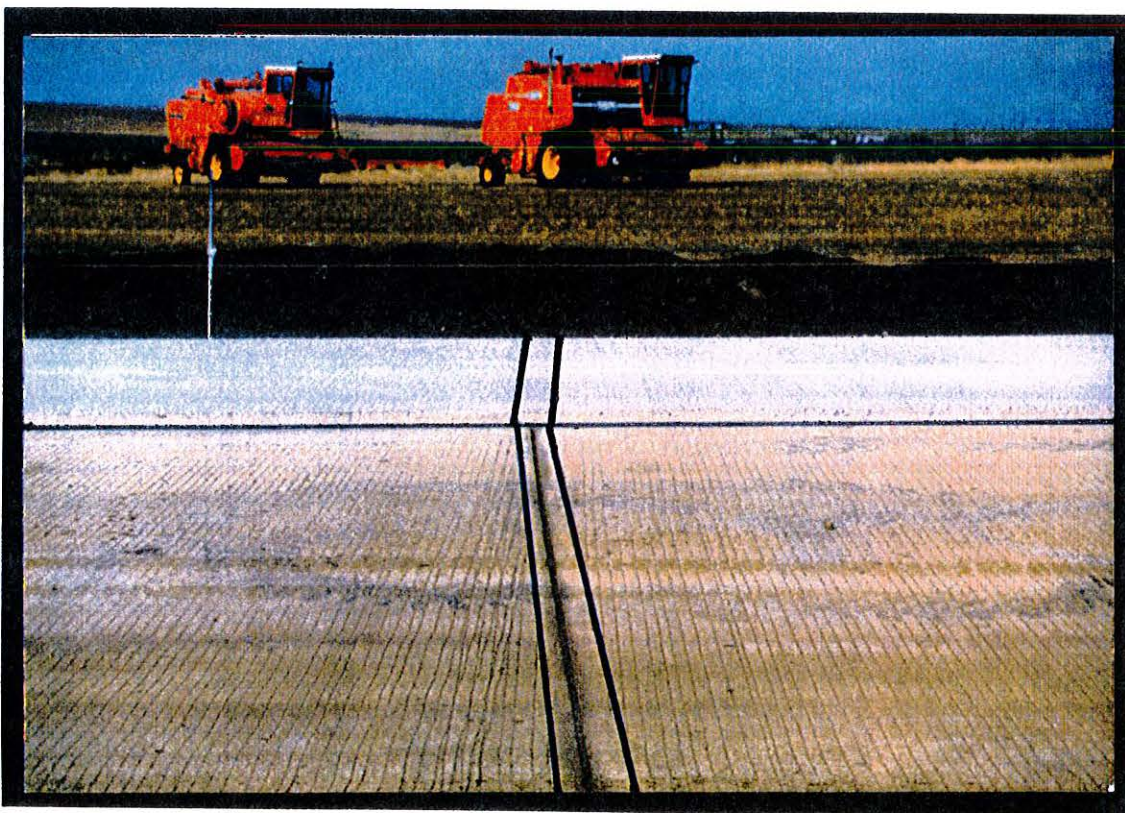
Figure 7 - Skewed Contraction Joint (With Respect To Adjoining & Center Line Joints)
