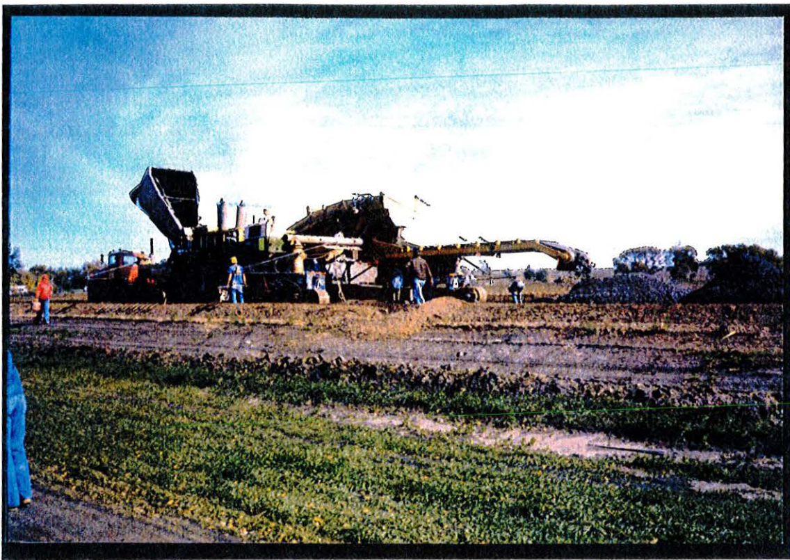
Figure 4 - Hopper and Conveyor Belt For Concrete Delivery
