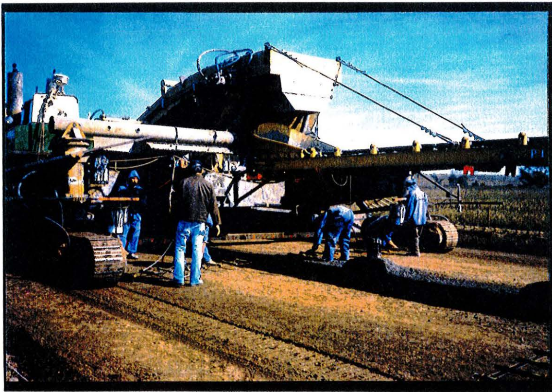
Figure 5 - Dowel Basket Installation Area (under conveyor belts)
