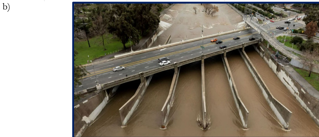
Figure 50. Long-tapered curtain wall efficiency: a) stress tests for CWLT; b) CWLT concept installed in Los Angeles River (Photo source: Ted Soqui/SIPA USA AP).
