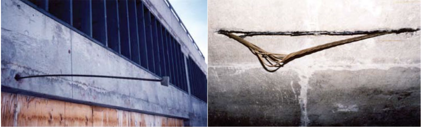
Figure 58. Erupted or ejected tendons from anchorage and slab soffit (Fallis et al. 45 )
