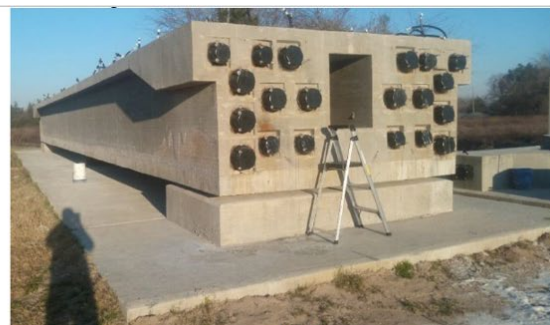
(e) Finished post-tensioned (U-beam) girder specimen
