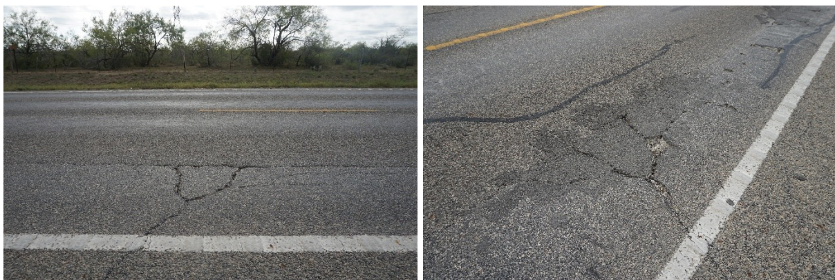
(a) Cracking Observed in 2019
