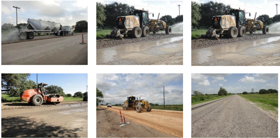
Figure 62. Construction Sequence on SH 202.
