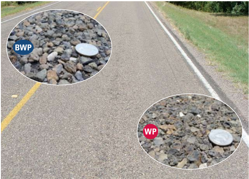
Figure 6. Lane with Slight Wheel Path Color Difference.
