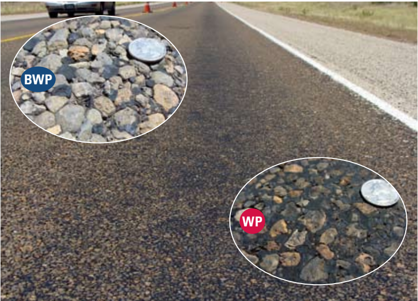
Figure 3. Lane with Moderate Flushing.
