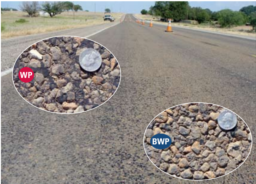
Figure 4. Lane with Mild to Moderate Flushing.
