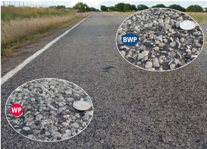
Figure 5. Lane with Mild Flushing.
