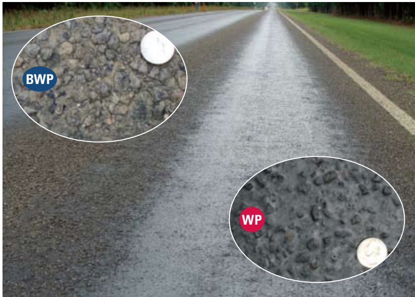
Figure 1. Lane with Severe Flushing.
