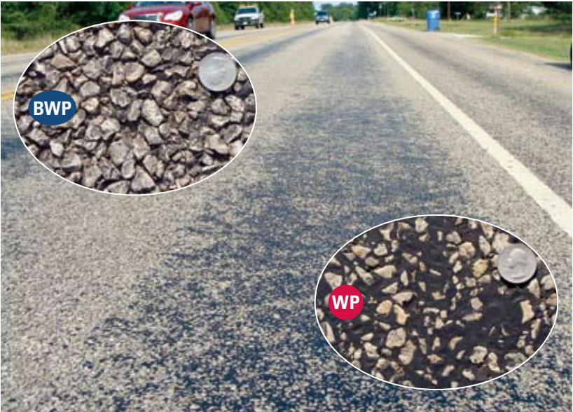
Figure 2. Lane with Moderate to Severe Flushing.
