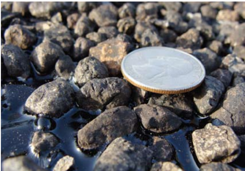
Figure 10. Wheel Path Aggregate Embedment Slightly Higher than Usually Desired after a Day or Two of Traffic.
