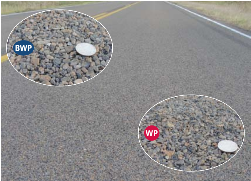
Figure 7. Lane with No Wheel Path Color Difference.
